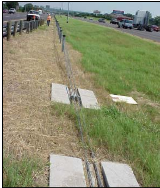
Figure 3-3. Good Example: Spacing between Cable Barrier and Metal Beam Guard Fence.
