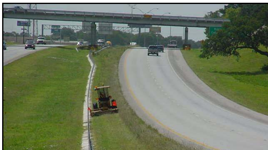
Figure 2-34. Concrete Mow Strip in Texas.
