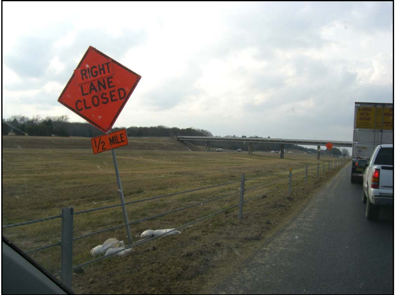
Figure 3-6. Example to Avoid: Shoulder Placement in Wide Median Creates Nuisance Hits.
