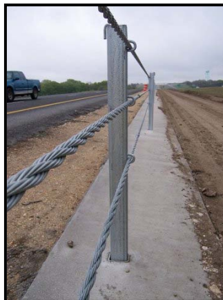
Figure 2-7. Gibraltar Cable Barrier System.
