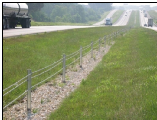
Figure 2-5. U.S. Low-Tension Cable Barrier System.
