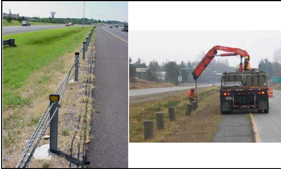
Figure 3-1. Posts in Concrete Drilled Shafts with Sockets.
