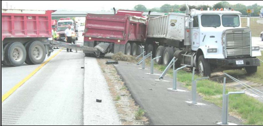
Figure 2-22. Successful Capture of Large Vehicles on I-20 in Parker County, TX.
