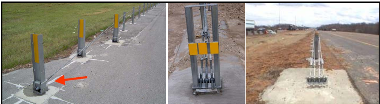
Figure 5-1. Cable Anchor Terminals (Left: Trinity/Nucor; Center: Gibraltar; and Right: Brifen).
