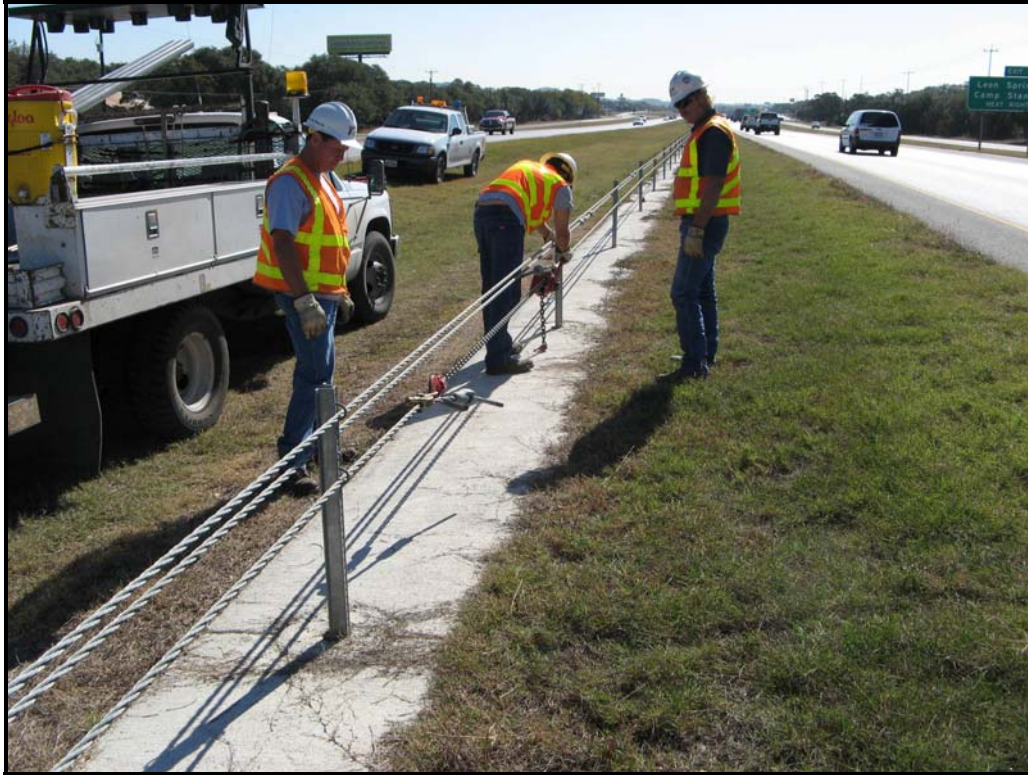
Figure 5-3. Simple Repair of Impact on IH 10 in Boerne.
