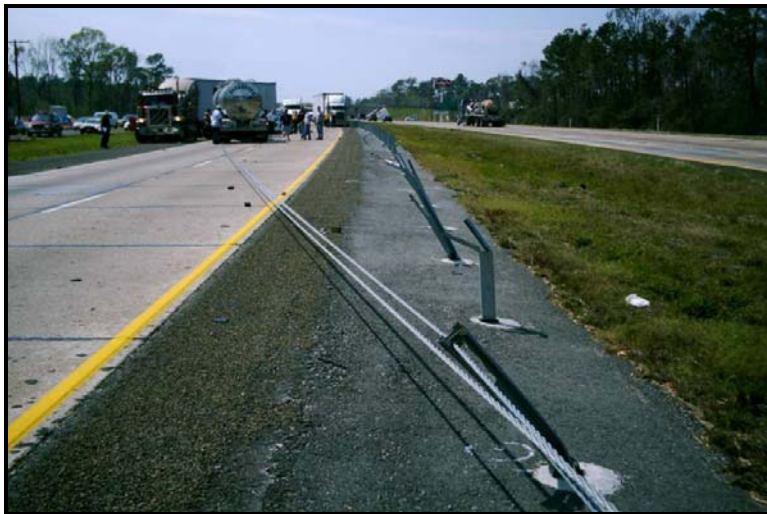
Figure 4-12. Example of a Semi-Tractor Trailer Cable Barrier Penetration Event.
