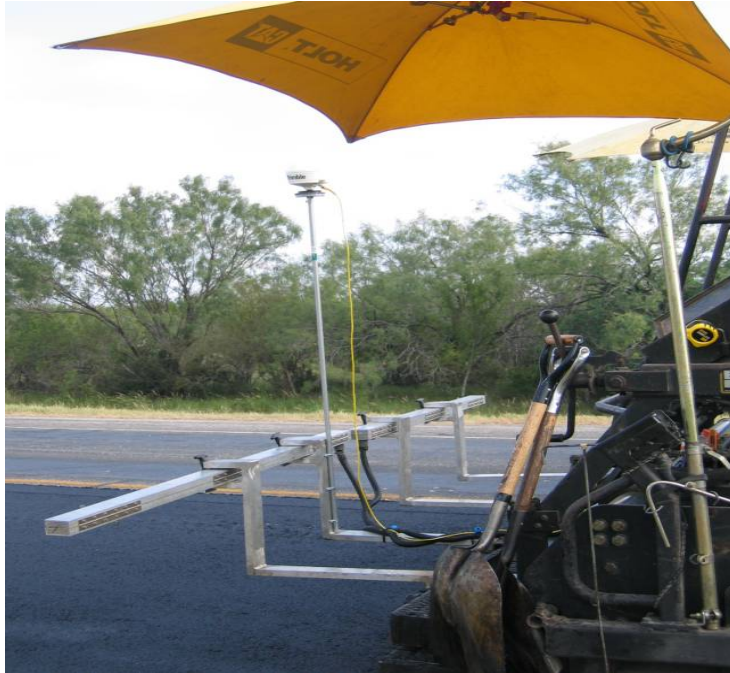
Figure 38. Infra-Red Monitoring of CAM Placement on US 90.
