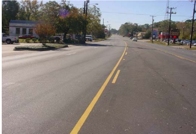
Figure 17. CAM Mix on US 59 Three Months after Placement.
