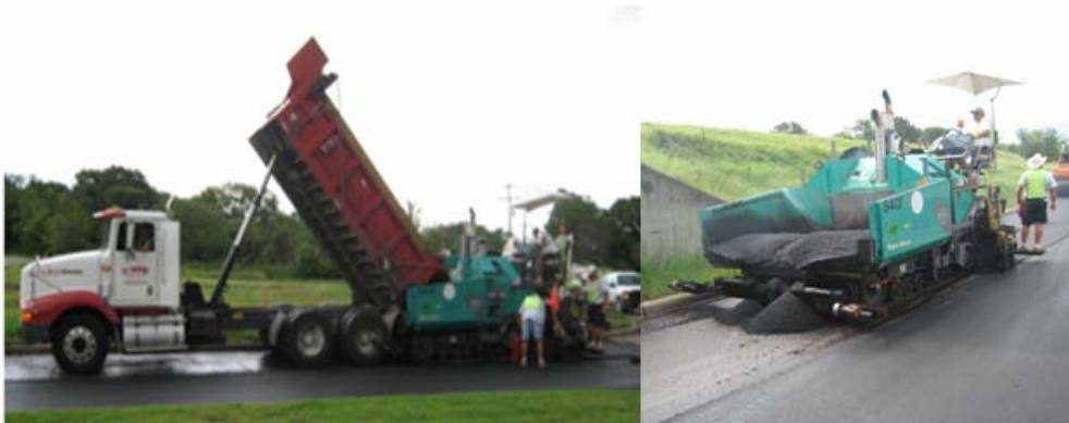
Figure 24. Paver Operation on the Pumphrey Drive, FTW.
