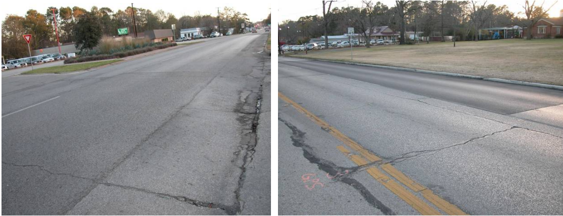
Figure 7. Location of Poor LTE on US 59 Prior to CAM Placement.
