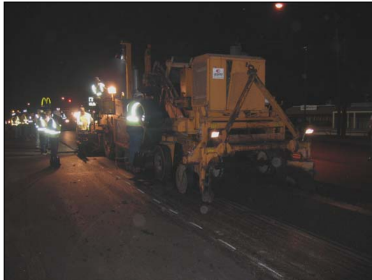
Figure 9. CAM Paving Operation on Business 59.
