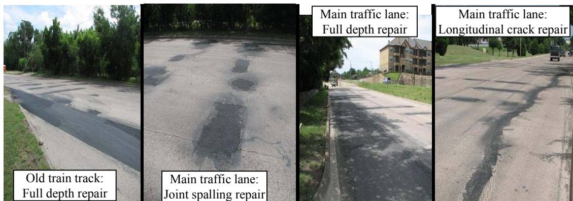
Figure 23. Repairs of Existing Distresses Before the HMA Overlay.
