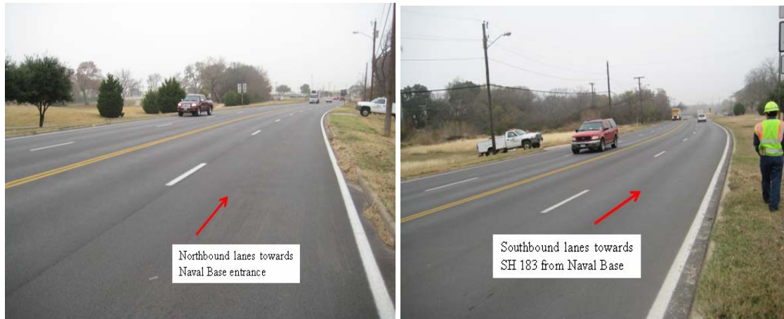
Figure 25. Overview on the Main Lanes between SH 183 and the Naval Base Entrance.
