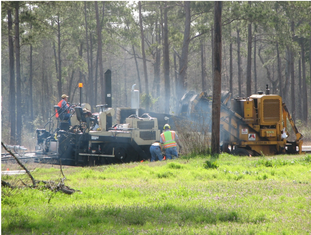
Figure 5.19. Construction of Lufkin WMA Field Trials.
