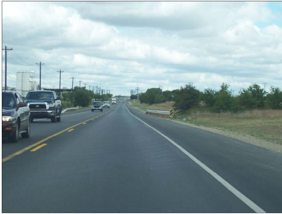
Figure 5.33. Fort Worth BU 287 WMA Project after One Year of Service.
