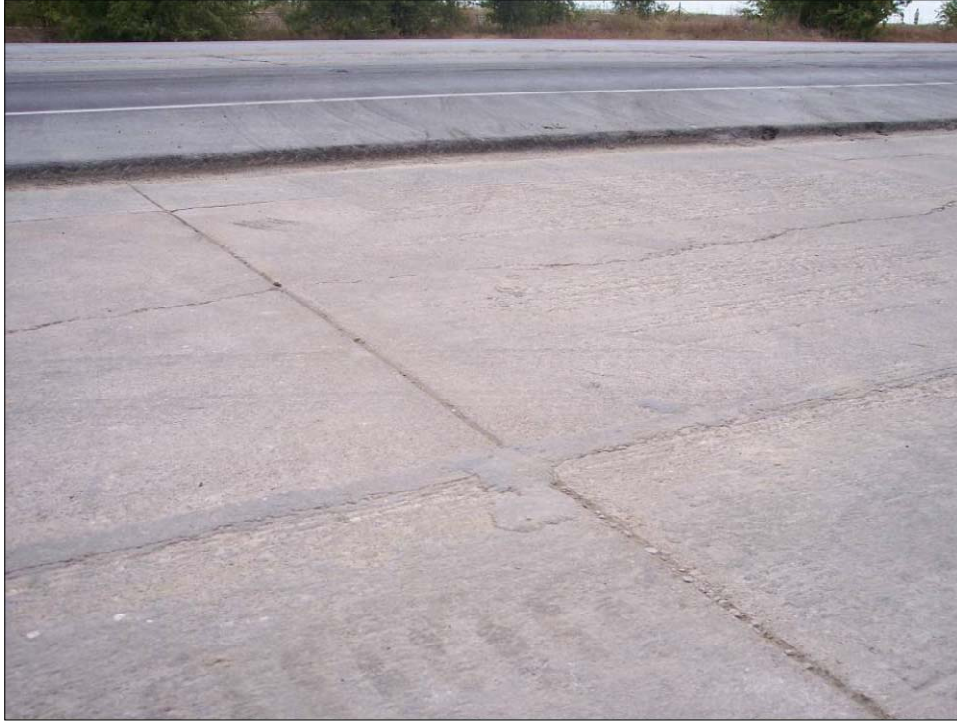
Figure 5.27. BU 287 Jointed Concrete Pavement Prior to Type D WMA Overlay.
