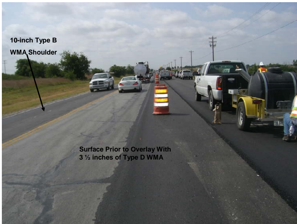
Figure 5.28. BU 287 Shoulder Rehab and Asphalt Pavement Prior to Overlay
