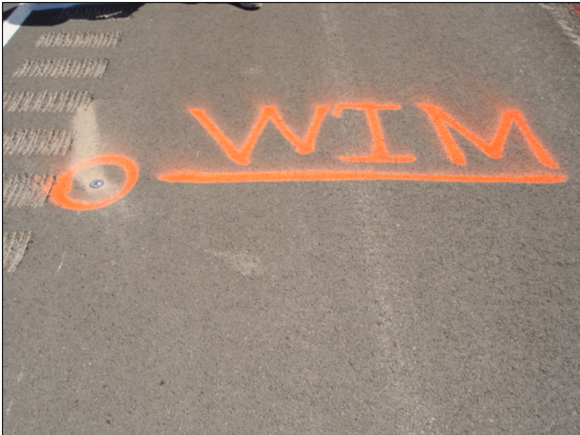
Figure E6. Marker Placed at Proposed Location of WIM Sensors on Eastbound Lanes.
