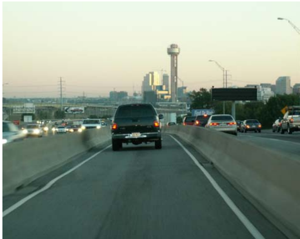
(a) Barrier-Separated HOV Lane on Northbound R.L. Thornton Freeway
