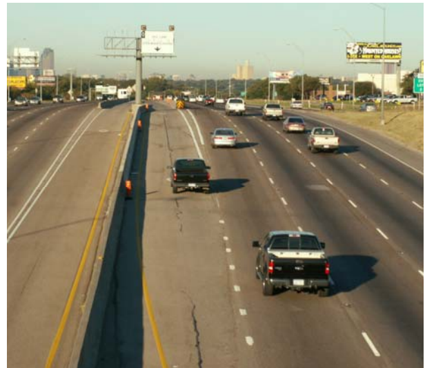
(b) Slip Ramp Access
