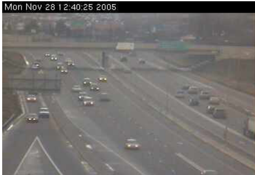
Figure 3-3. HOT Lane Access Point on I-394 EB at US-169, Minneapolis, MN. (Image courtesy of Minnesota DOT)
