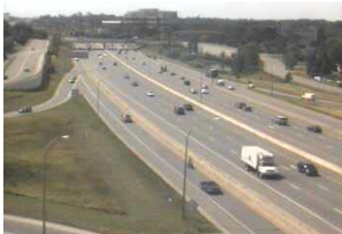
Figure 3-15. Image from MnDOT Camera on I-394 EB at US-169, Minneapolis, MN ( 19 ).
