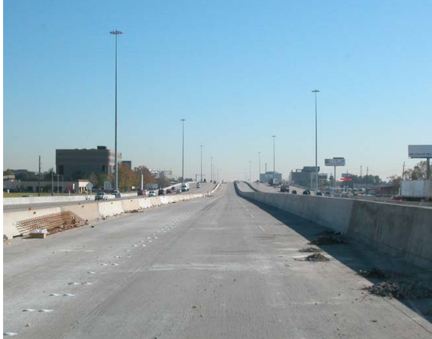
Figure 3-7. Closed Median Area on I-10 Near Sites 4 and 5.
