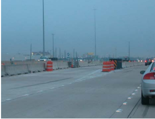
(a) Entrance to Barrier-Separated HOV Lane on Katy Freeway
