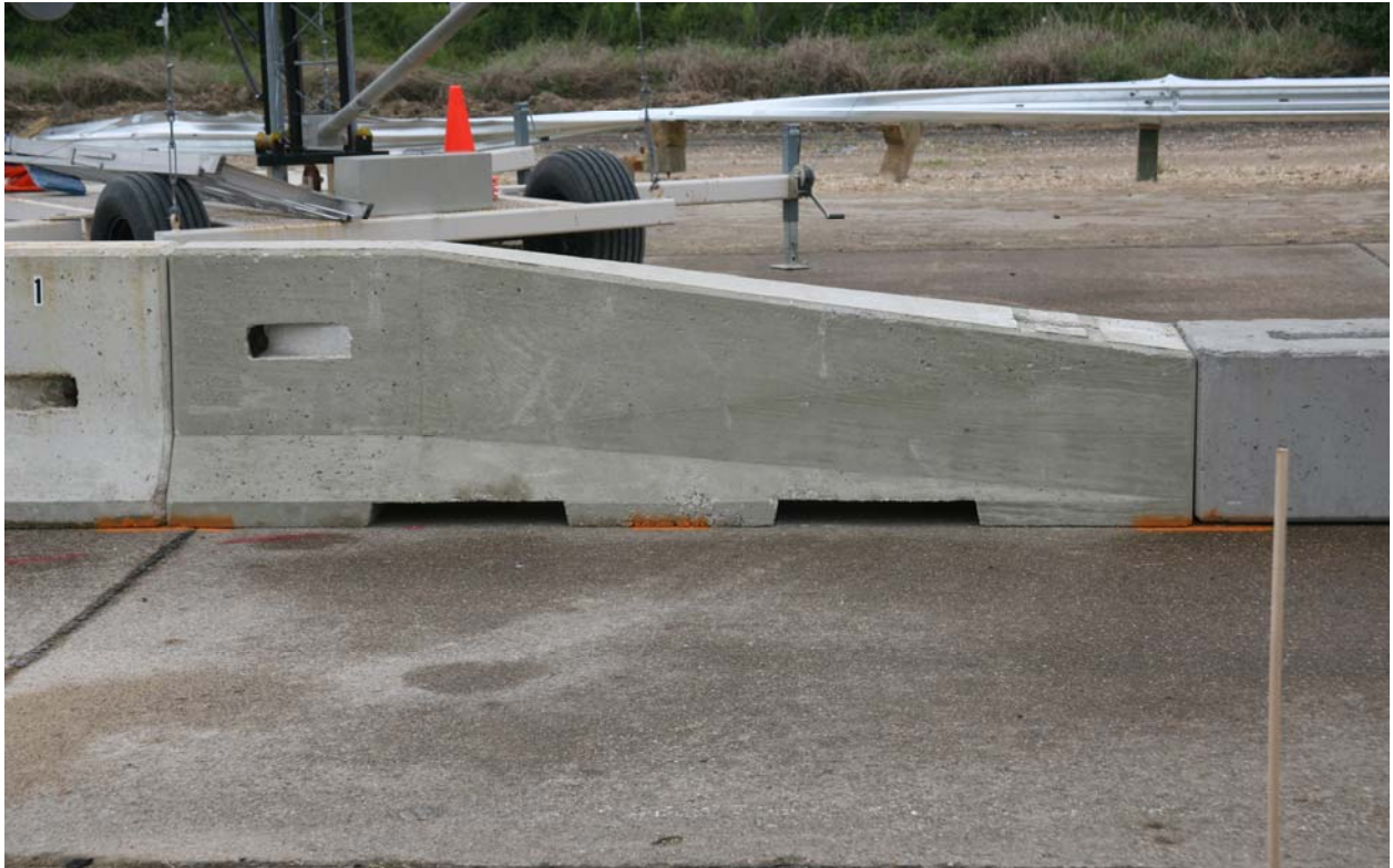
Figure 14. Low-Profile Transition Installation before Testing.
