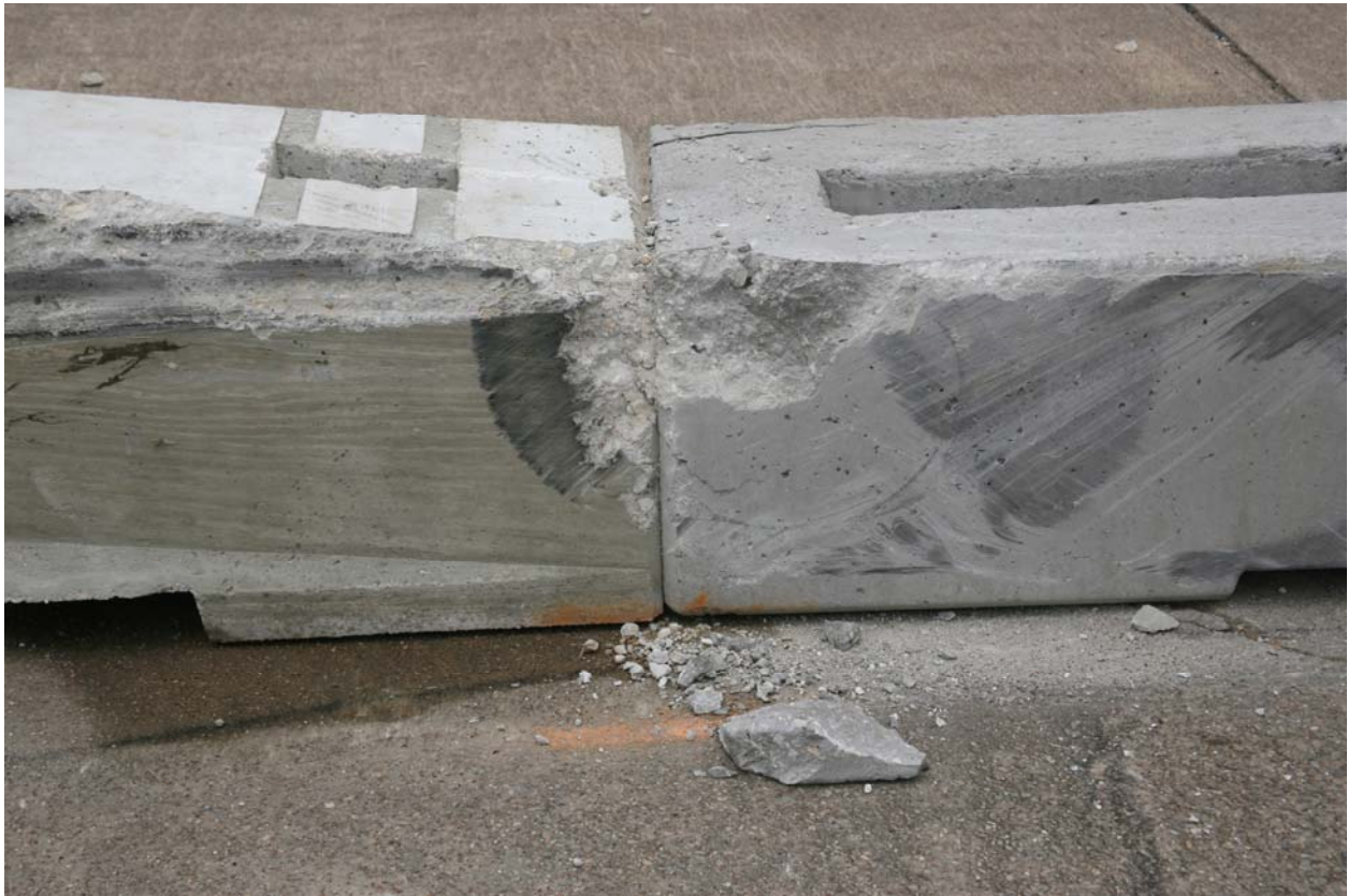
Figure 18. Installation after Test No. 455276-1.
