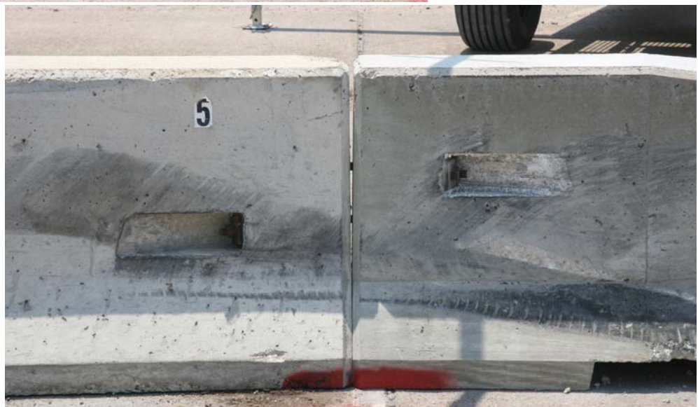
Figure 25. Installation after Test No. 455276-2.
