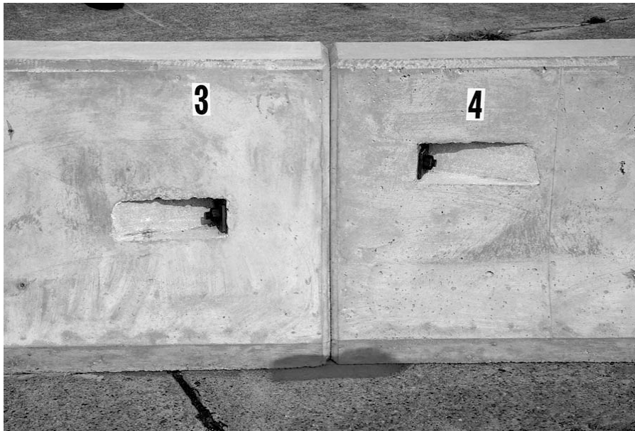
Figure 3-5. F-Shape Concrete Safety Barrier with X-Bolt Connection.
