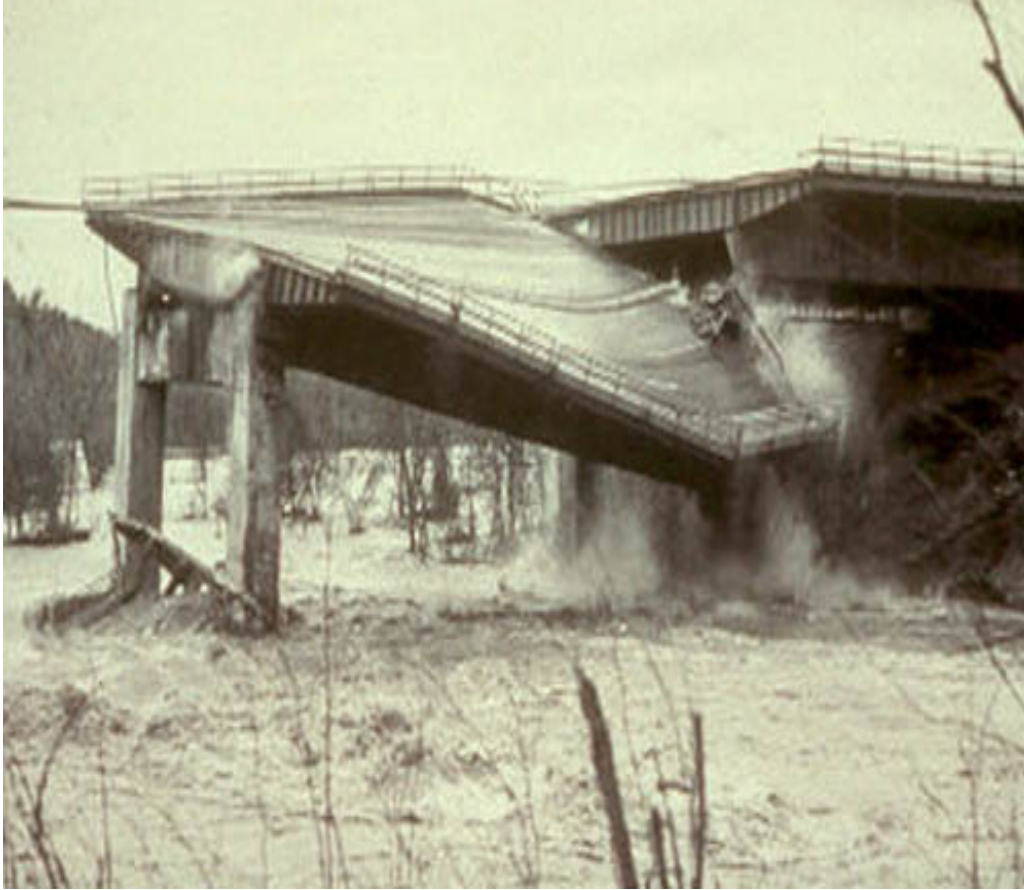
Figure 8-5. One of the Schoharie Creek Bridge Spans Plunging into the River.
