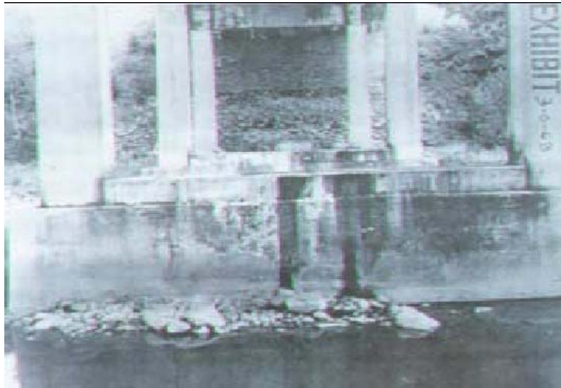
Figure 8-9. Photo of Pier 2 Taken in 1977.
