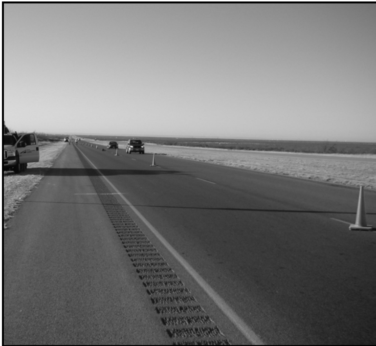
Figure 40. CMHB-F Pavement Containing Type II Tire Rubber – US 385, Odessa.
