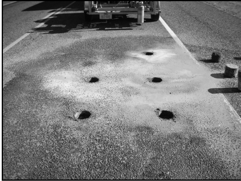
Figure 21. Typical Coring Layout at Section with HMA Layer (SH 176 in Odessa).
