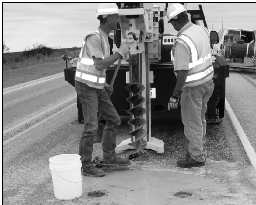
Figure 22. TTI Auger Used to Obtain Flexible Base and Subgrade Samples.
