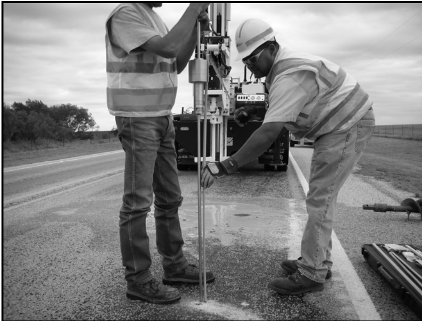
Figure 18. DCP Testing in Outer Wheel Path.
