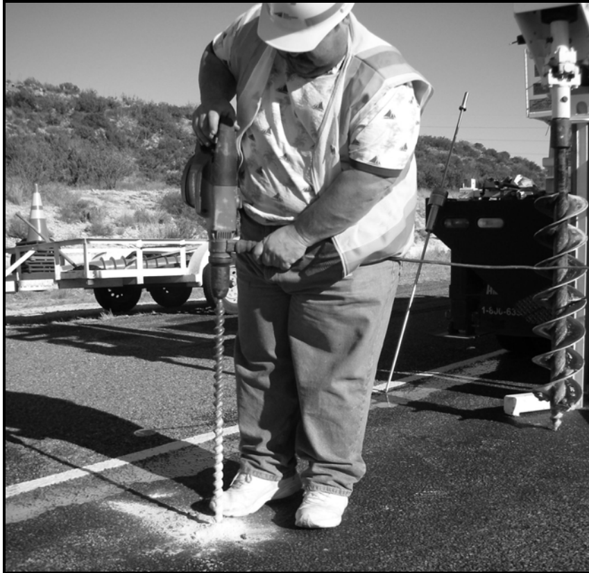
Figure 17. Drilling Asphalt Mixture before DCP Testing.
