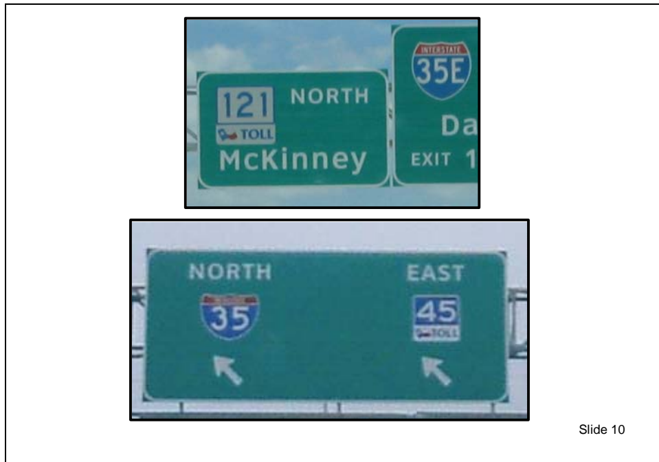
Figure 7. Comparison of Toll Route Marker Background Color for Applications on Green Guide Signs.
