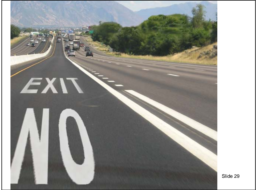
Figure 19. Managed Lane Ingress Only Area Using Text with No Passing Zone Lane Line Treatments.
