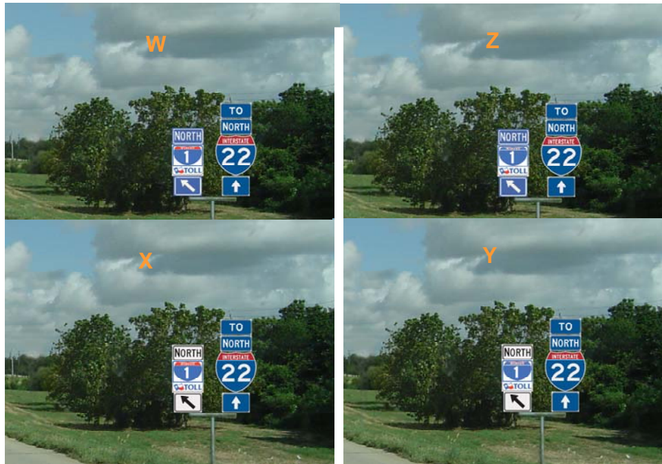
Figure 9. Toll Route Markers for an Interstate Toll Road Entrance Ramp Next to a Trailblazer Sign for an Adjacent Interstate.
