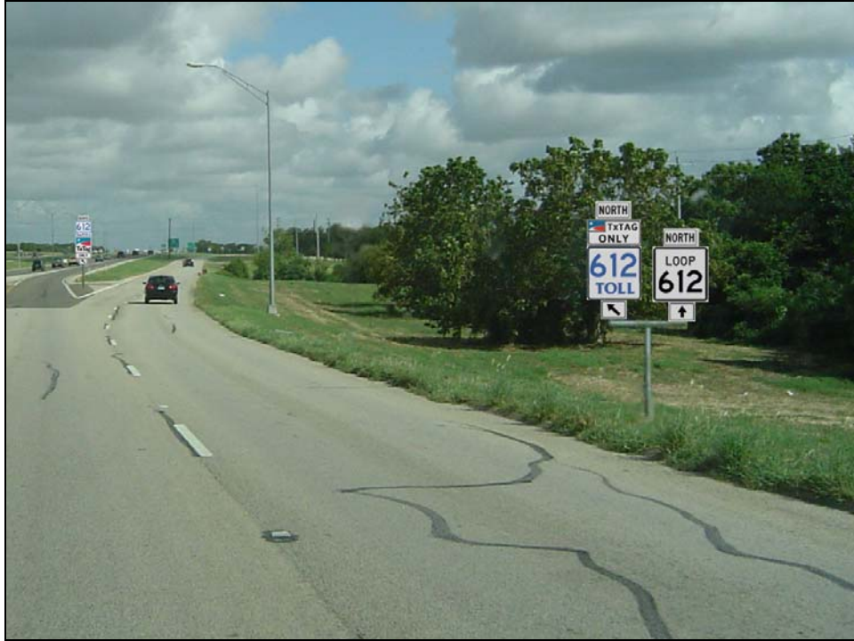
Figure 5. Modified Route Marker for a Toll Road Entrance Ramp from a Non-Toll Frontage Road.
