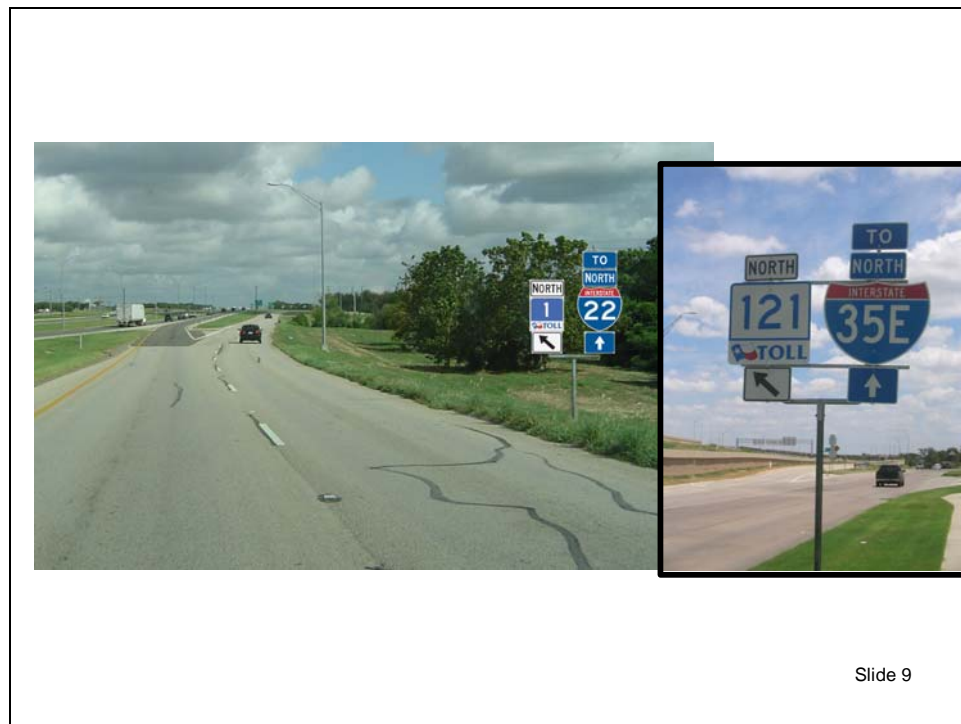
Figure 6. Toll Route Markers Compared to Interstate Route Markers.
