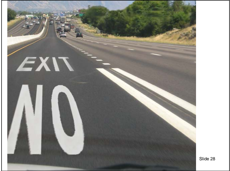
Figure 18. Managed Lane Ingress Only Area Using Text with Conventional Lane Line Treatments.
