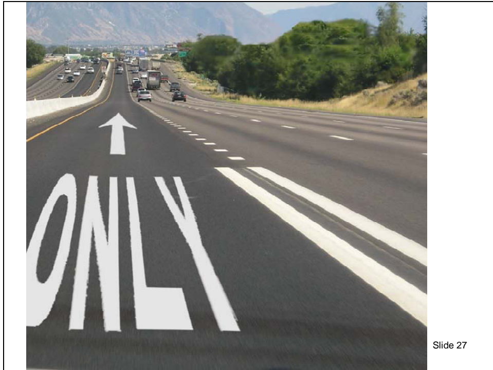
Figure 17. Managed Lane Ingress Only Area Using Text and Arrow with Conventional Lane Line Treatments.
