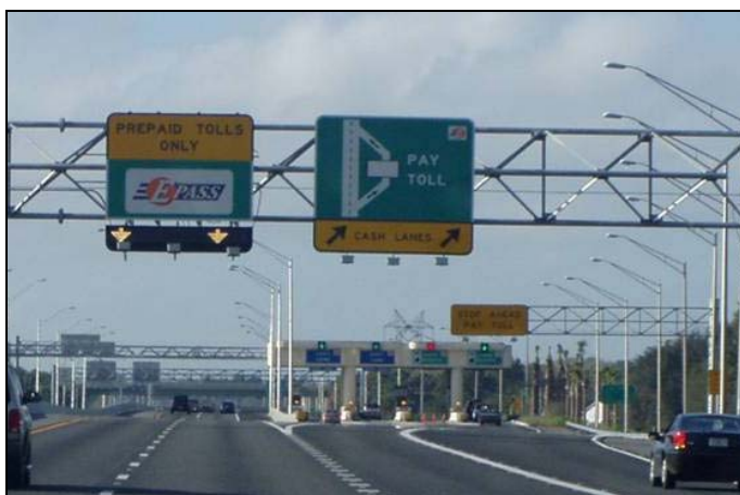
Figure 5. Colorado E470 Cash Pull-Out Lanes. (photo courtesy of Wilbur Smith Associates)
