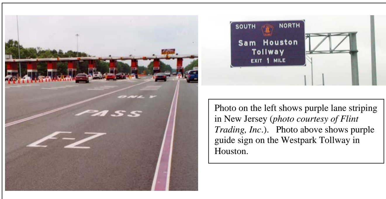
Figure 3. Use of Purple for Markings and Signs for Toll Facilities.
