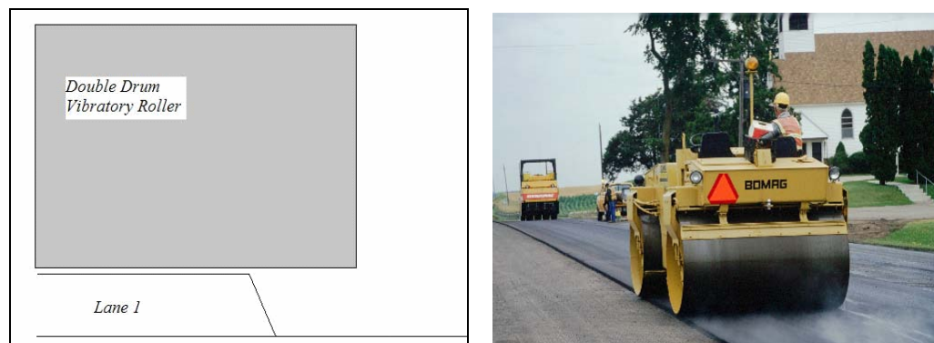
Figure 18. Proper Location of the Steel Wheel Roller over the Unsupported Edge of the First Paved Lane (Scherozman 2004)
