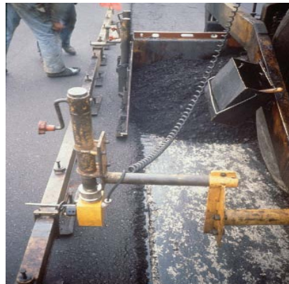
Figure 20. Proper Amount of Overlap from Lane 2 to Lane 1 (Scherozman 2004)
