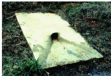
Figure 13. Outlet Pipe Headwall (Baumgardner 2002)
