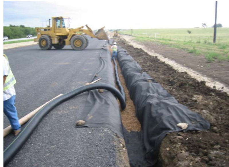
Figure 9. Typical Edge Drain Configuration at the Shoulder's Edge (Scullion, 1998)
