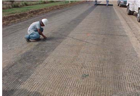
a. Geogrid Being Placed on OSR
