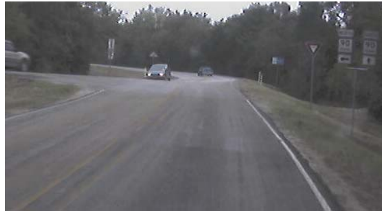
Figure 15. Flexible Pavement with Steep Side Slopes
