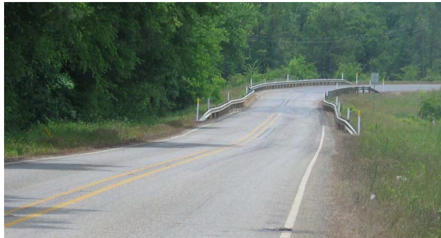
Figure 17. Flexible Pavement Widening at Narrow Bridge Approach
