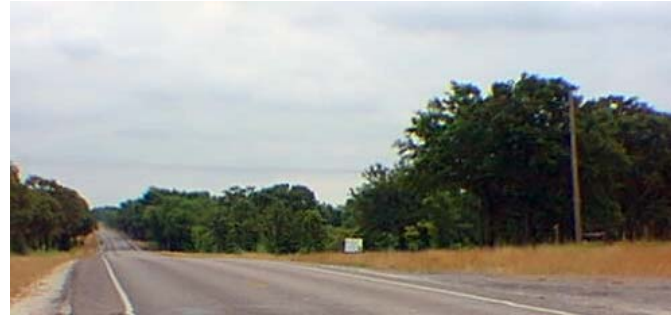
b. OSR after 2 Years of Geogrid Placement
