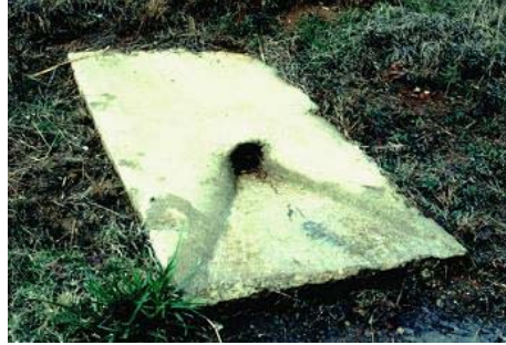
Figure 7. Outlet Pipe Headwall (Baumgardner 2002).
