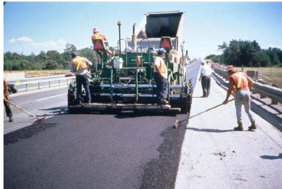
Figure 15. Improper Raking of the Longitudinal Joint (Scherozman 2004).
