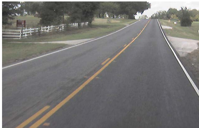
Figure 26. Flexible Pavement Section in Good Condition.
