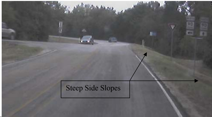
Figure 4: Flexible Pavement with Steep Side Slopes
