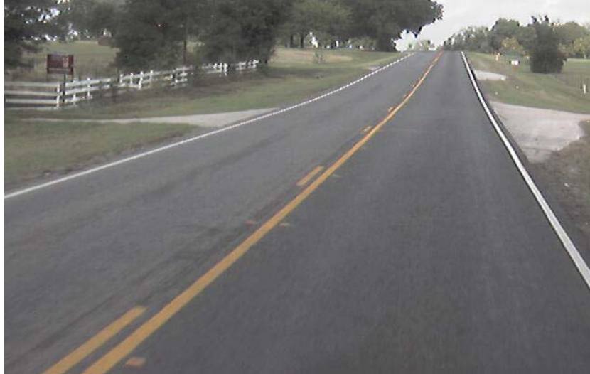
Figure 1: Flexible Pavement Section in Good Condition
