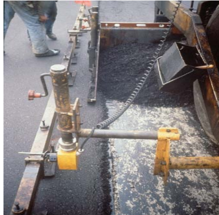
Figure 14. Proper Amount of Overlap from Lane 2 to Lane 1 (Scherozman 2004).
