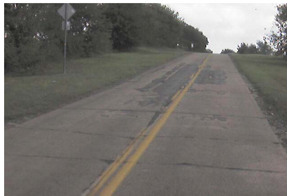
Figure 32. Jointed Concrete Pavement.
