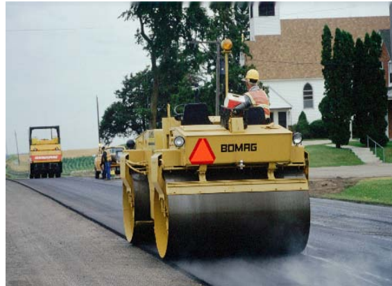
Figure 12. Proper Location of the Steel Wheel Roller over the Unsupported Edge of the First Paved Lane (Scherozman 2004).
