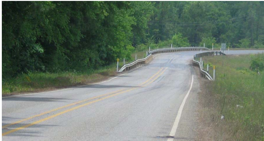
Figure 5: Narrow Bridge Approach
