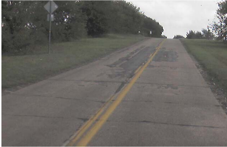
Figure 3: Jointed Concrete Pavement
