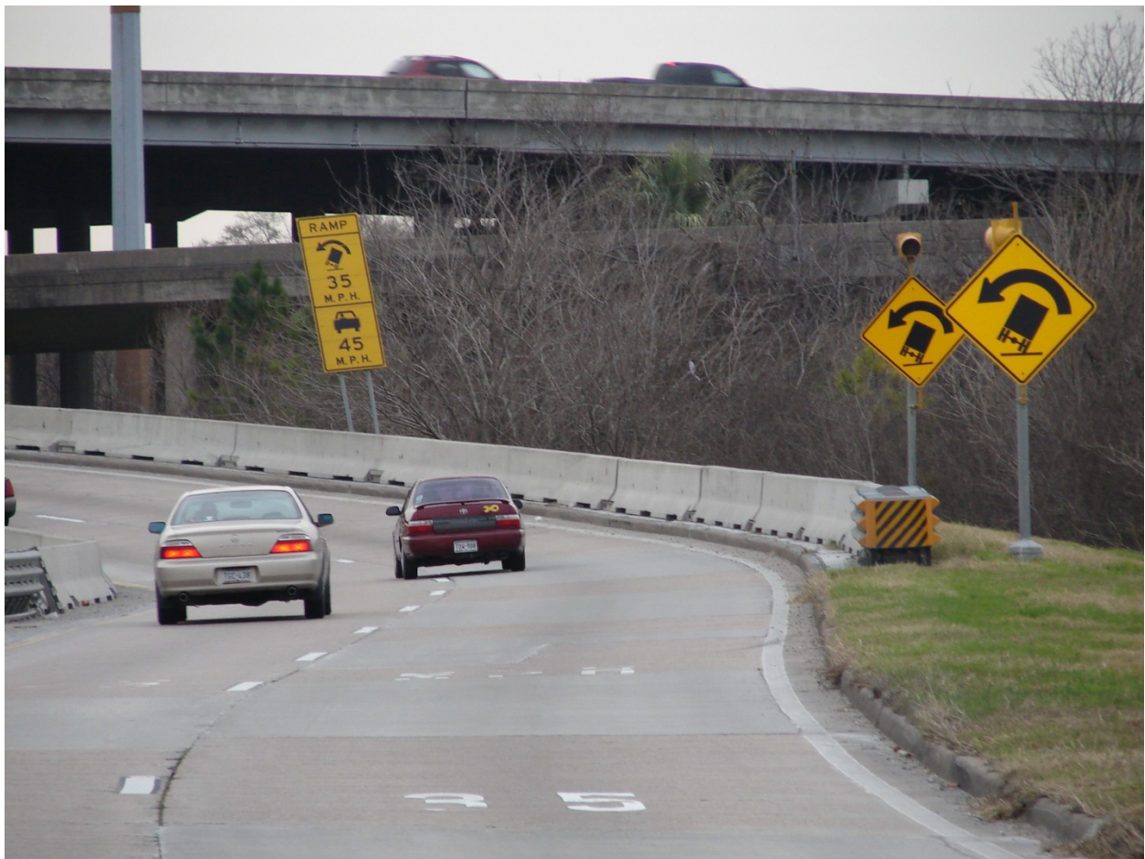
Figure 12. Active Curve Warning System. (Photo courtesy of TTI)
