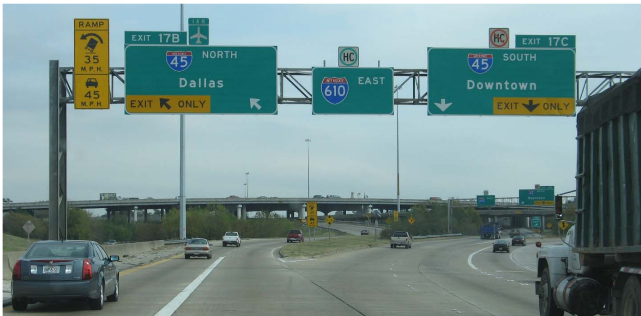
Figure 7. Dual Speed Warning Sign for Trucks – Gantry Mounted. (Photo courtesy of TTI)
