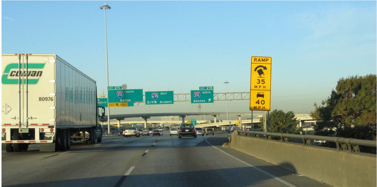
Figure 8. Dual Speed Warning Signs for Trucks – Ground Mounted. (Photo courtesy of TTI)
