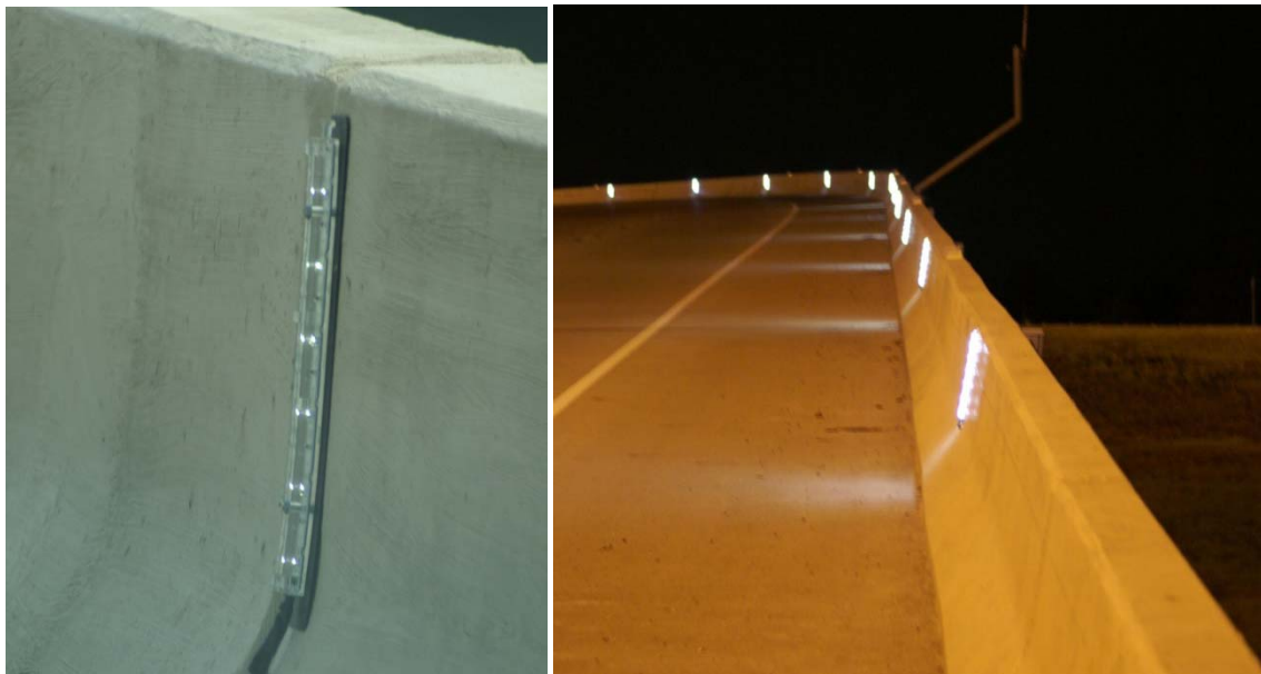
Figure 10. Curve Warning Barrier Markings. (Photo courtesy of TTI)
