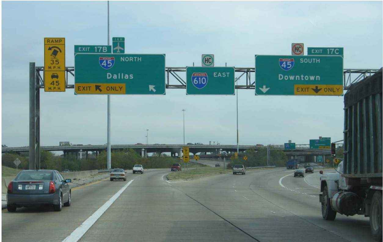
Figure 7. Dual Speed Warning Sign for Trucks – Gantry Mounted. (Photo courtesy of TTI)
