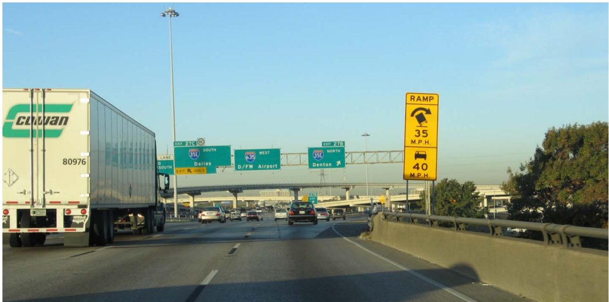
Figure 8. Dual Speed Warning Signs for Trucks – Ground Mounted. (Photo courtesy of TTI)
