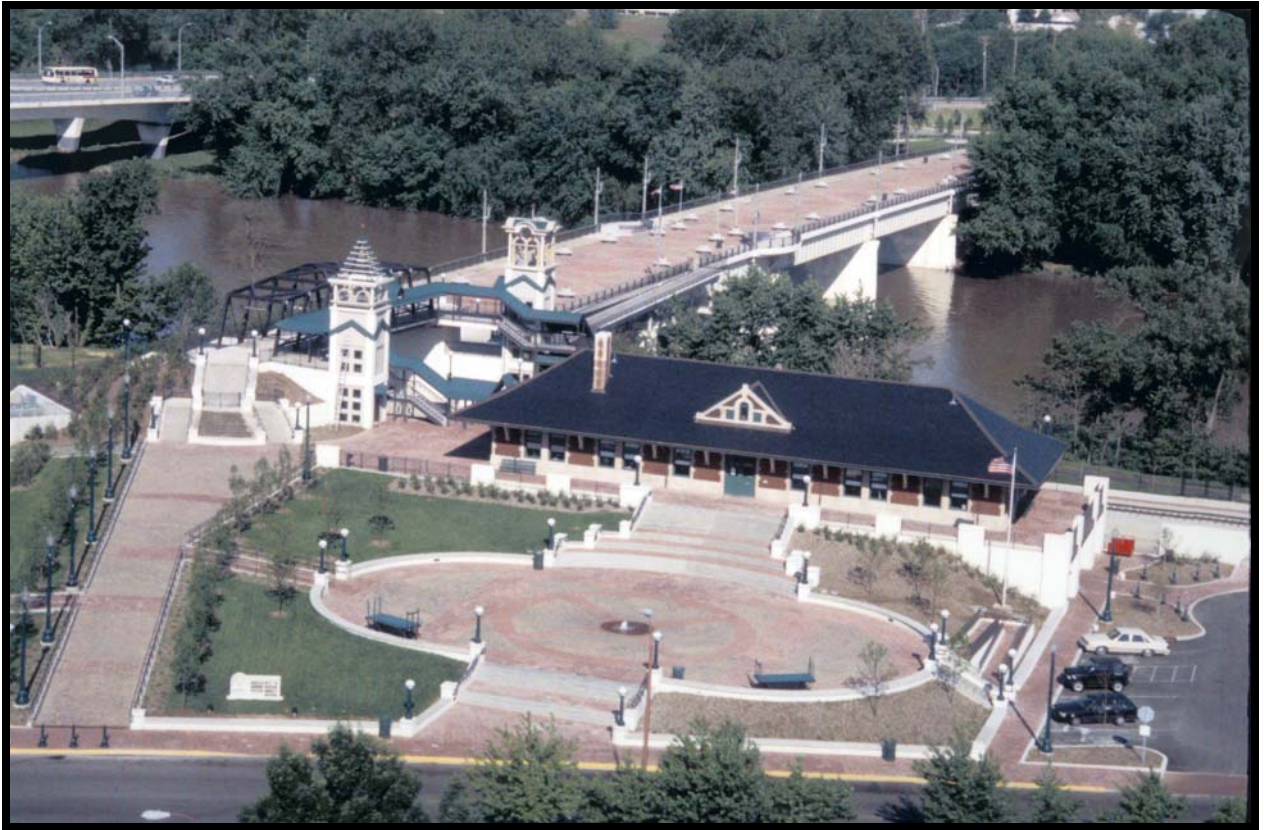
Figure 17. Relocated and Restored Lafayette Big Four Station/Riehle Plaza/Pedestrian Bridge Area
