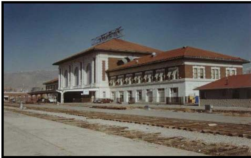
Figure 34. Rio Grande Depot Rail Yard Prior to Redevelopment.
