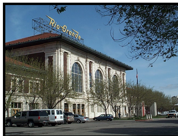
Figure 29. Rio Grande Depot.
