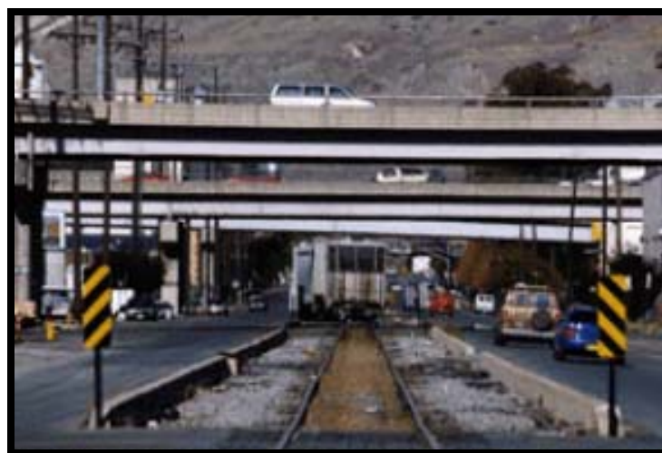
Figure 31. Viaducts at the 400 West Spur (41).
