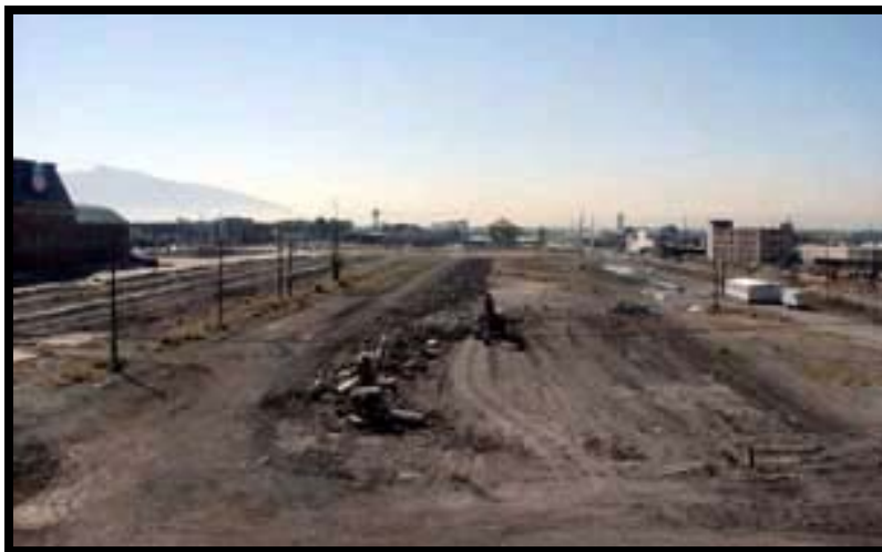
Figure 33. Union Pacific South Yard and Vicinity Prior to Redevelopment.
