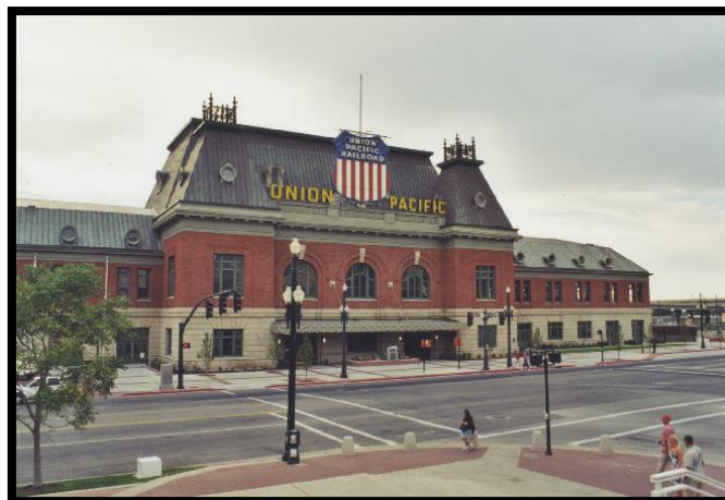
Figure 28. Restored Union Pacific Depot.
