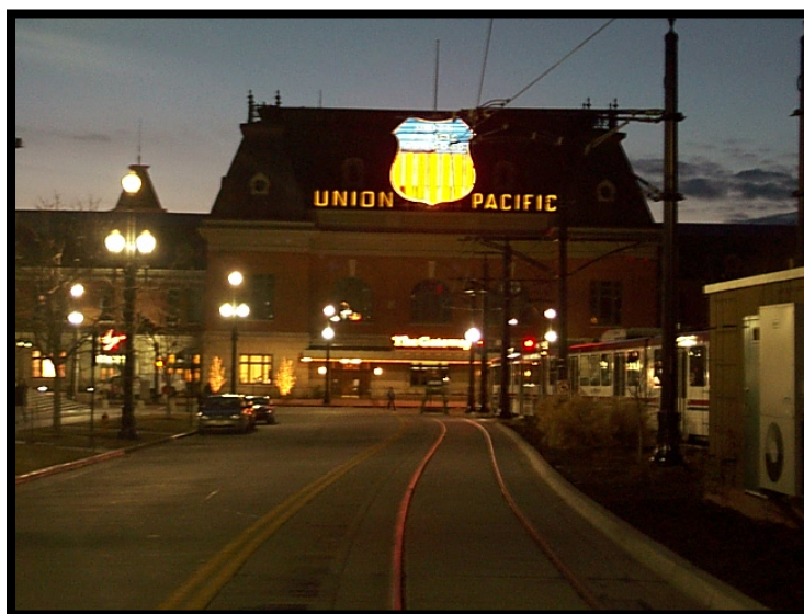
Figure 36. Light Rail at the Union Pacific Depot.
