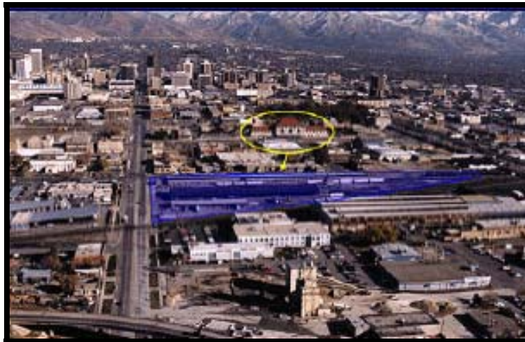
Figure 32. Site of the Multimodal Hub in Relation to the Rio Grande Depot (41).
