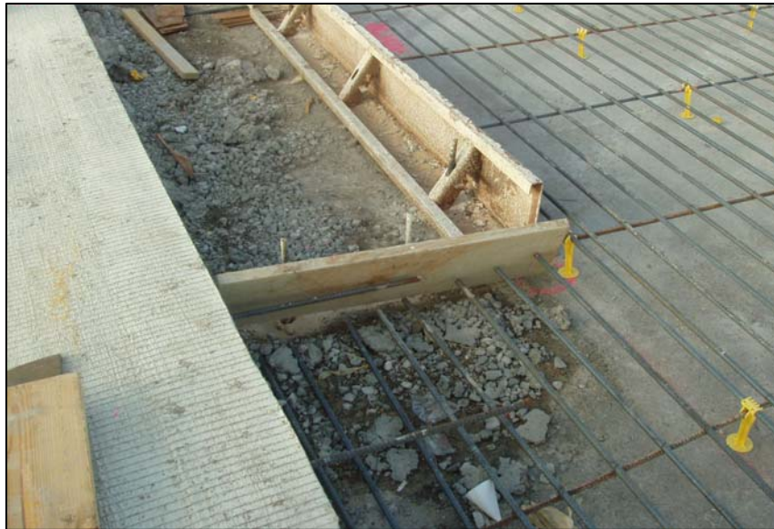
Figure 3-16 Gore Area in the Ramp Transition.
