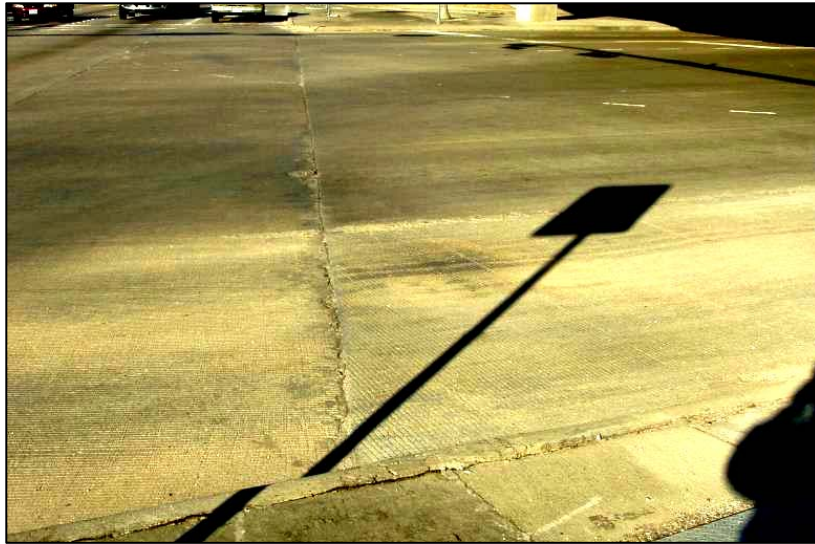
Figure 3-8 Good Performing Longitudinal Construction Joint.
