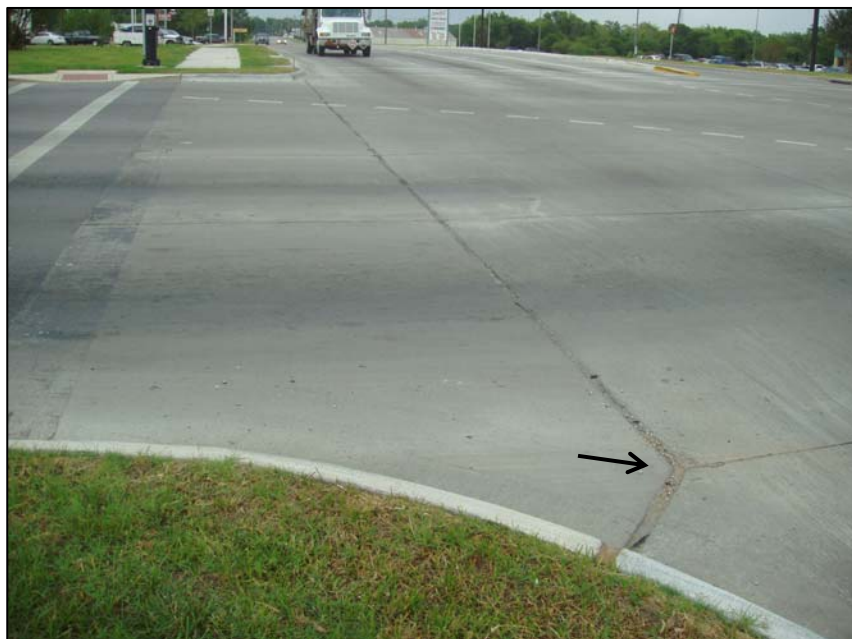
Figure 3-15 Obtuse Angle Joint Corner in the Intersection.
