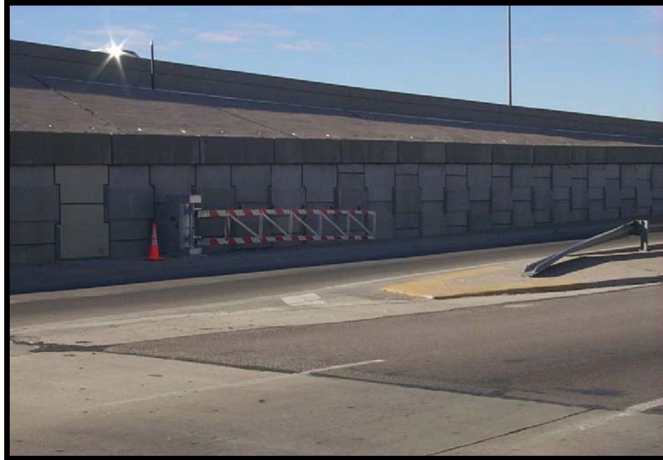
Figure 3. IH-10 Ramp Closure – El Paso, TX.
