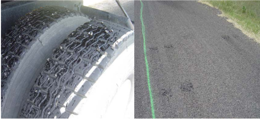
Figure 28. Low Level of Damage.
