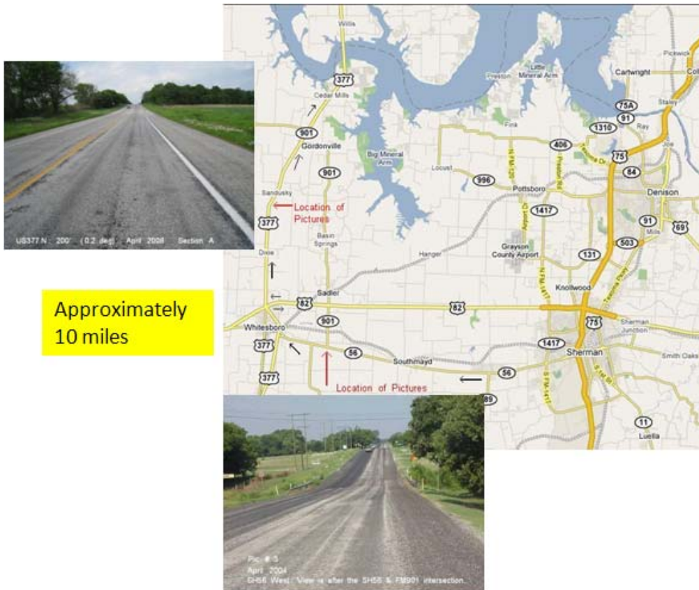
Figure 9. SH56 and US377 Seal Coat Damaged Sections.
