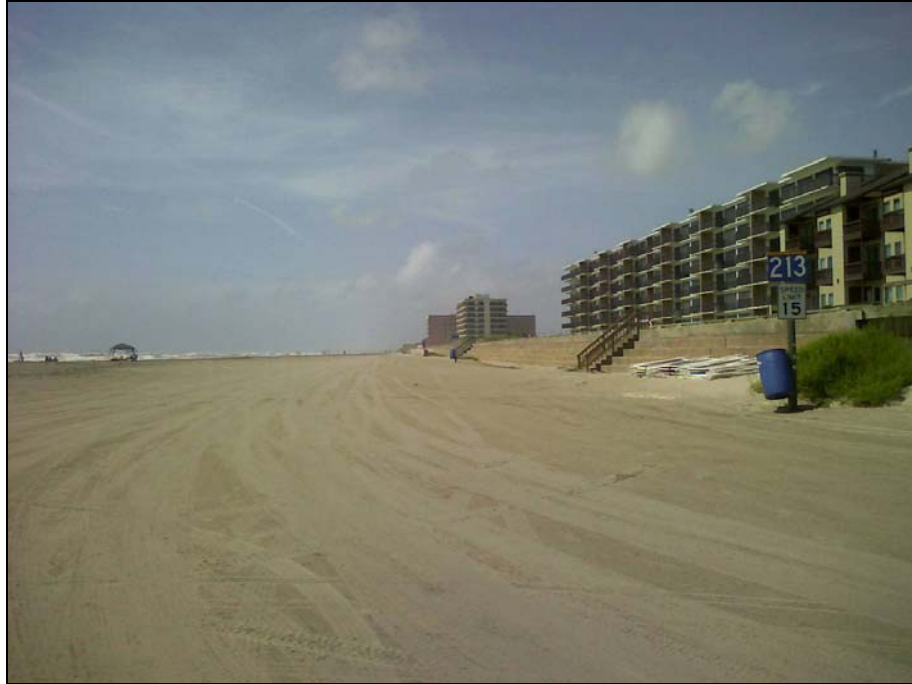
Figure 38. Photograph of Site 7, Showing Proximity to Hotels and Other Developments.
