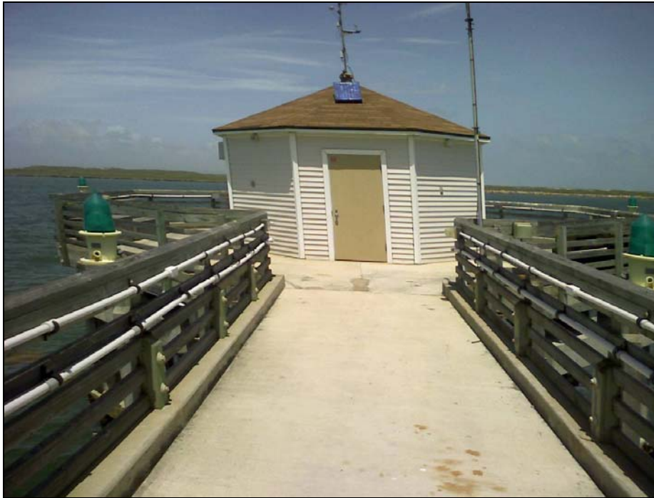
Figure 39. Photograph of Two-Level Pier at UTMSI Site.
