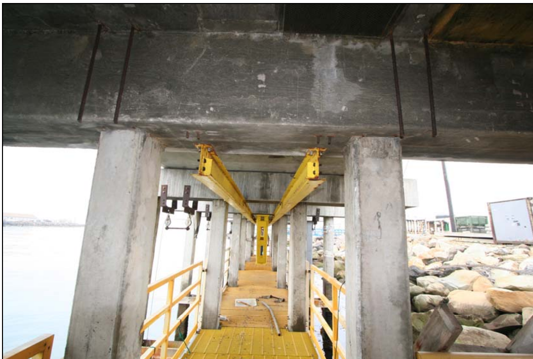
Figure 32. Pier Substructure with Access Structure.
