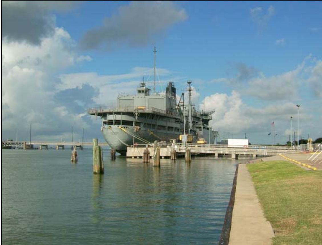
Figure 42. Docking Facilities on Pelican Island and Causeway to Galveston.
