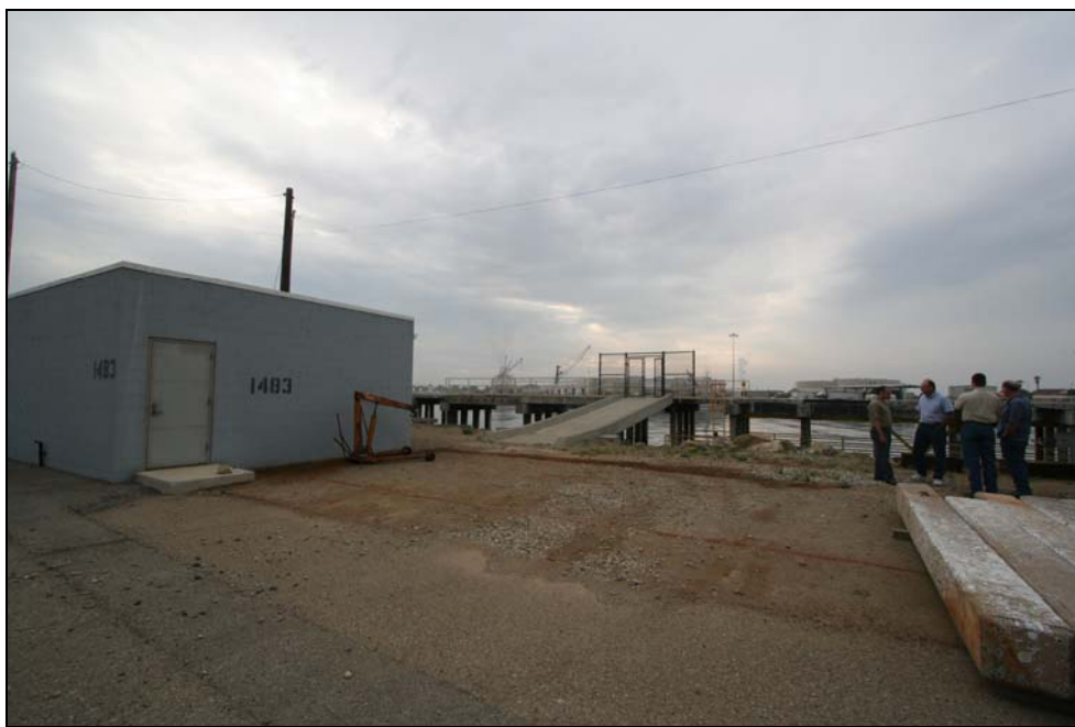
Figure 31. Storage Building and Area near the Access to the Facility.
