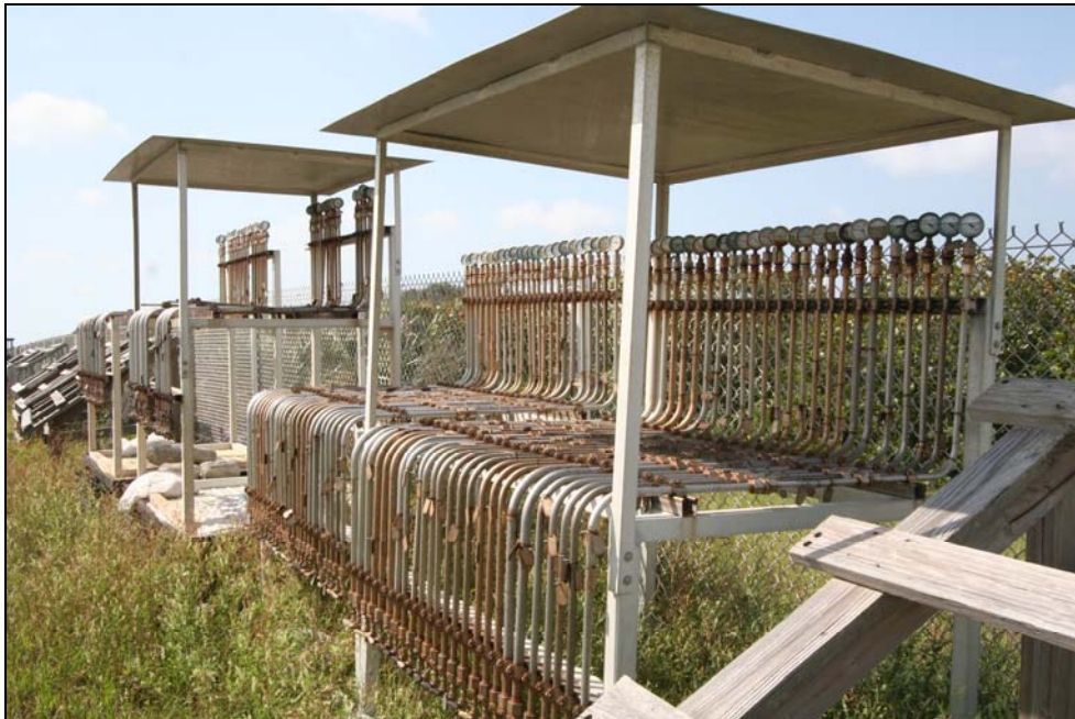
Figure IV.2. Piping under Exposure.
