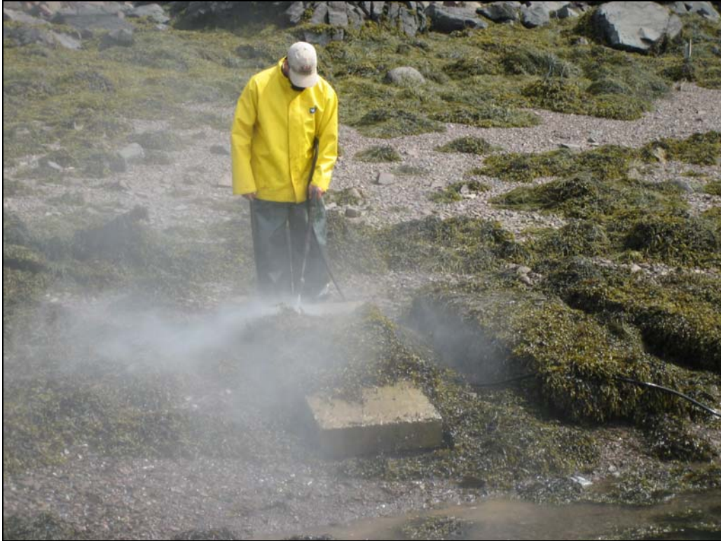
Figure IV.8. High-Pressure Washing with Water.
