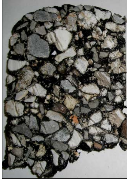
Figure 32. Aggregate Breakage Due to Compaction (I-35-PG Mixture).
