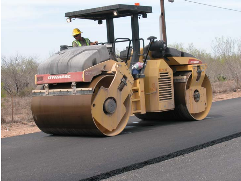
Figure 3-2. Finish Roller on FM 649.
