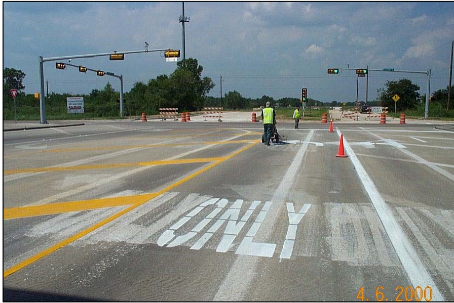
Figure 43. Pavement Marking Obliteration by Grinding.
