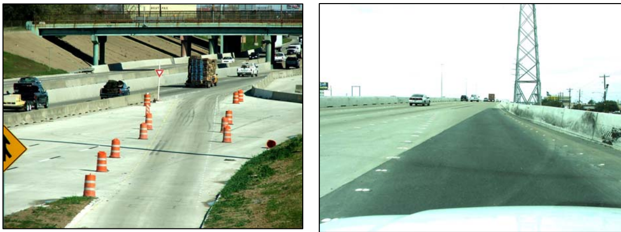
Figure 15. Examples of Removal or Reductions in Acceleration Lane Lengths.
