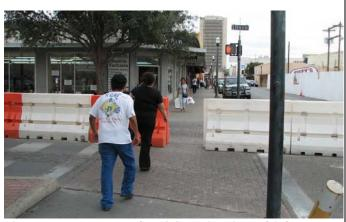
Figure 4-18. Example of Opening in Vehicle Barricade
