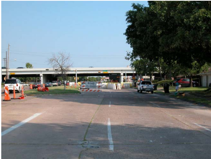
Figure 5. US-59 at Fondren, Looking West.
