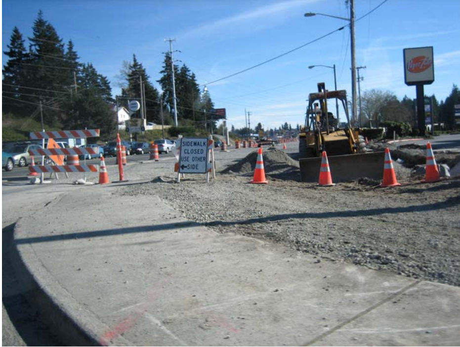
Figure 22. Sidewalk Closed with Visible Construction in Path.
