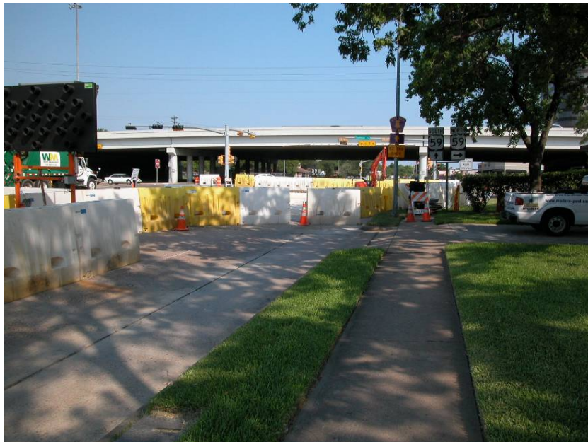
Figure 6. Sidewalk Closed on Fondren.
