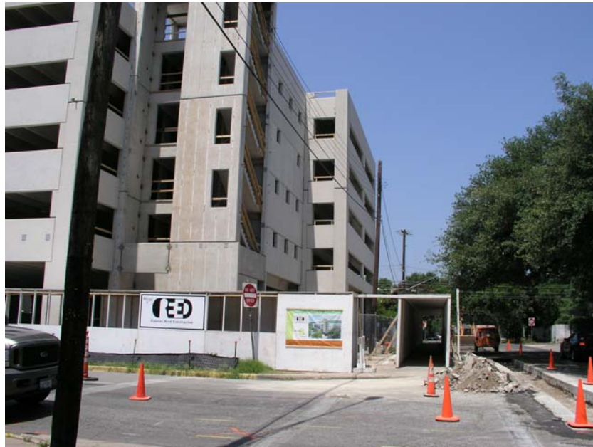
Figure 3. Parking Garage Construction in Austin.
