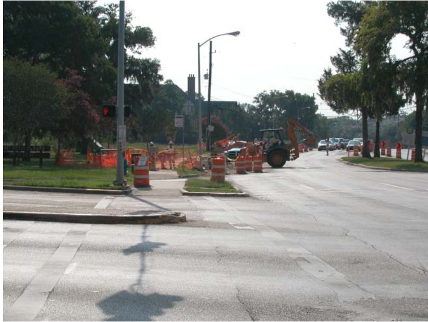
Figure 7. Holcombe at Braeswood, Looking East.
