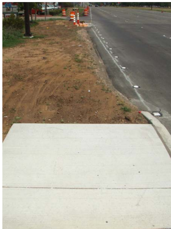
Figure 16. Pathway Paving Removed.
