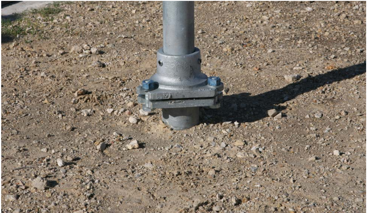
Figure 3.3. Test Article/Installation before Test 452108-1 and 2.
