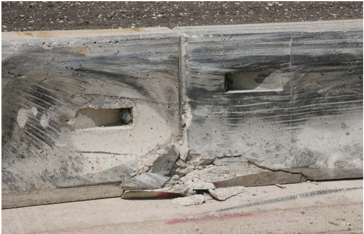
Figure 22. Installation after Test No. 452106-4.
