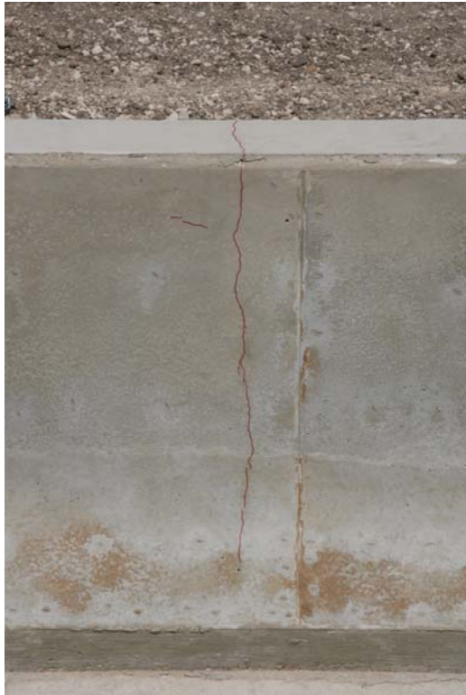
Figure 10. Installation after Test No. 452106-3.
