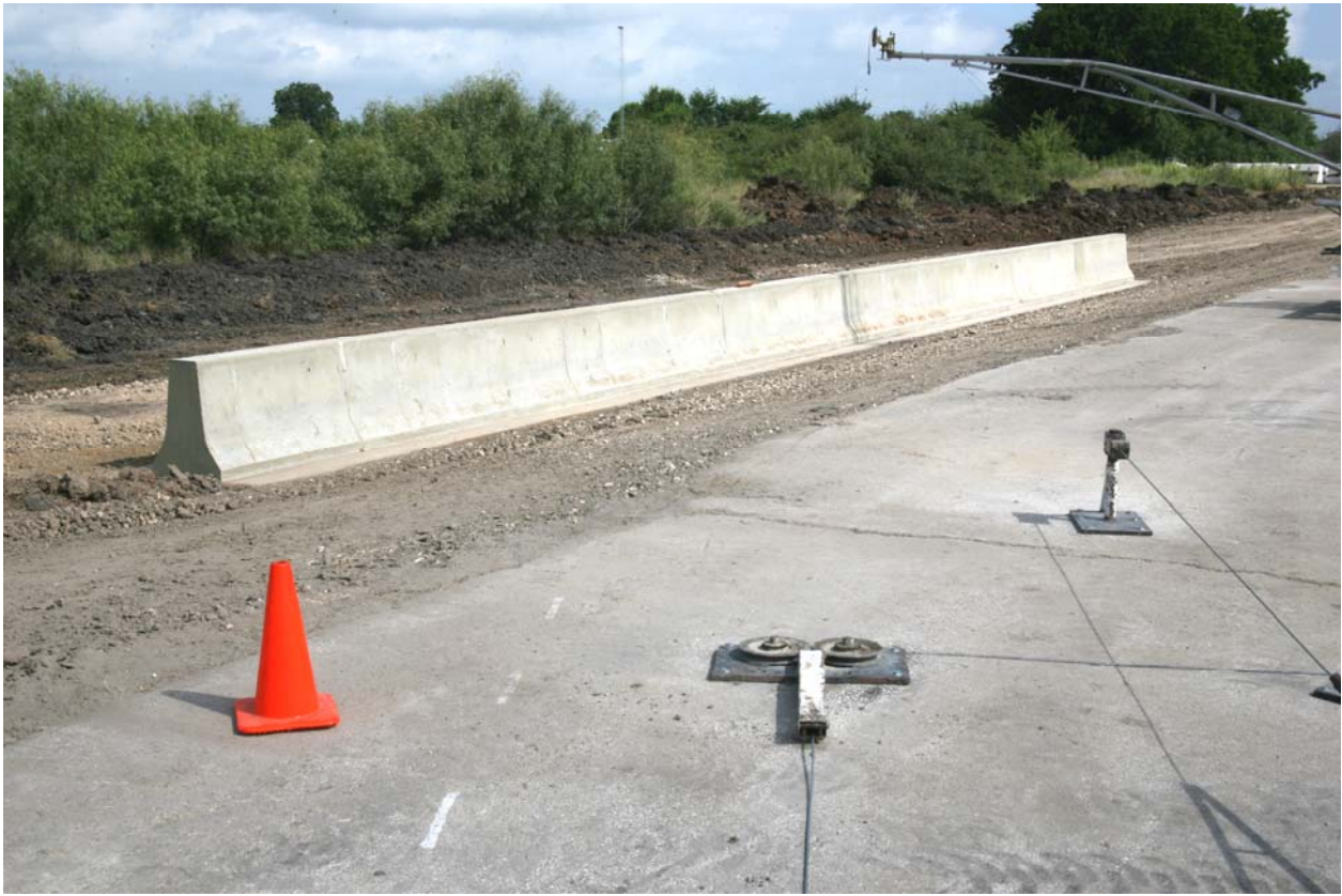
Figure 6. Permanent F-Shape Barrier on 6V:1H Slope before Test No. 452106-3.
