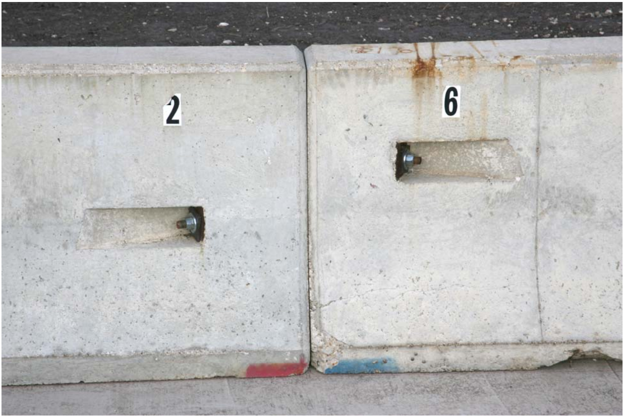
Figure 18. Free-Standing, Precast F-Shape Barrier on 6H:1V Slope before Test No. 452106-4.
