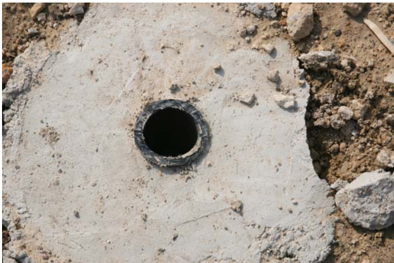
Figure 13. Installation after Test No. 452106-2.
