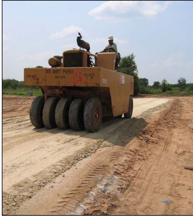
Figure 1.16. Rolling with the Pneumatic on the Groesbeck Test Site.
