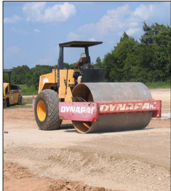
Figure 1.13. Rolling at Spicewood Test Site.
