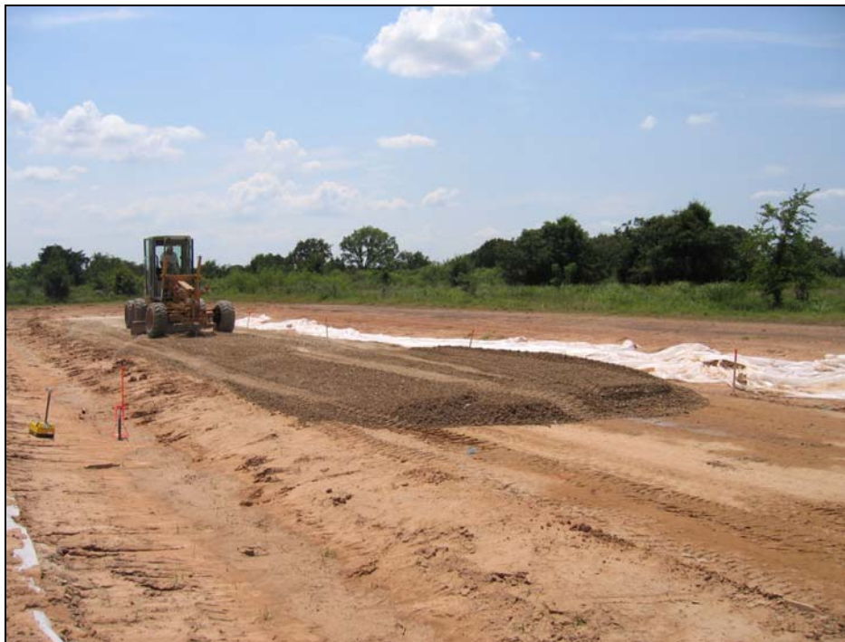
Figure 1.12. Spreading Spicewood Base at Test Site.
