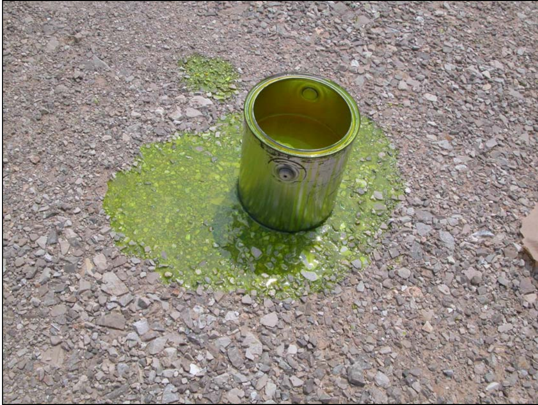
Figure 4.5. Epofix Epoxy with Fluorescent Dye Placed on Base Material.
