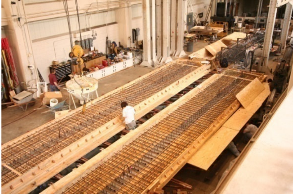
Figure 4.19. Placement of Reinforcement.
