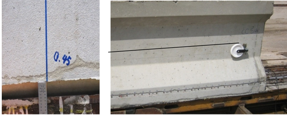
(a) (b) Figure 4.38. Initial Camber Reading (a) and Stringlines (b).
