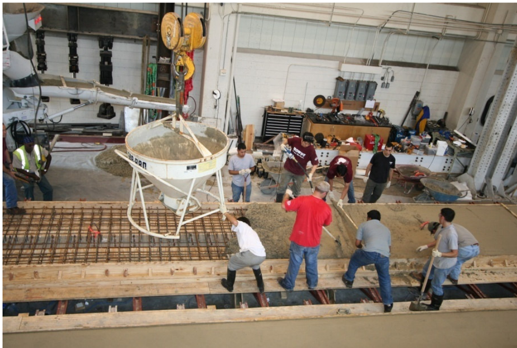
Figure 4.20. Placement of Deck Concrete.
