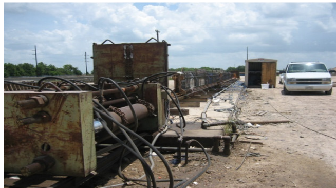
Figure 4.17. Prestressing Bed with Strands.
