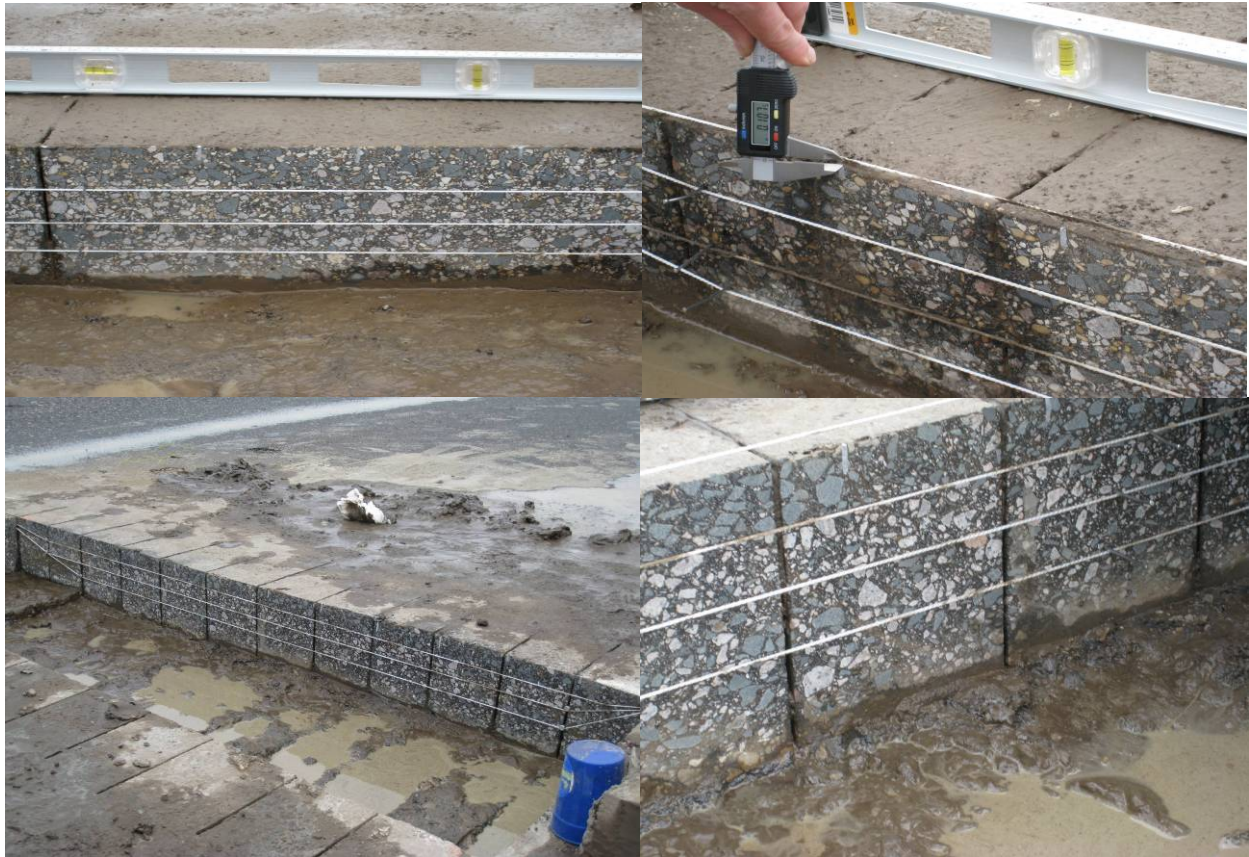
Figure 3-2. Trench Wire Lines for Overlay Sections 508 (Top) and 507 (Bottom) on US175.
