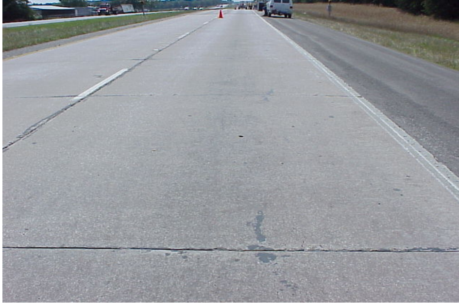
Figure 29. In-situ Conditions of Reversal Deflection Site on US82 (12).
