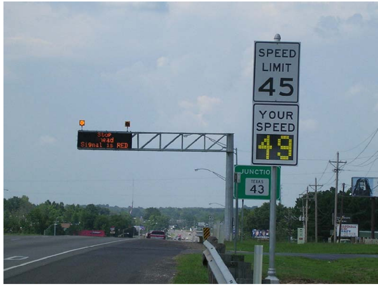
Figure 10. Overhead Electronic Matrix Sign.
