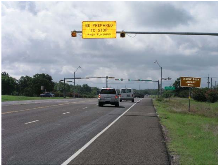
Figure 5. Overhead AWEGS Sign.
