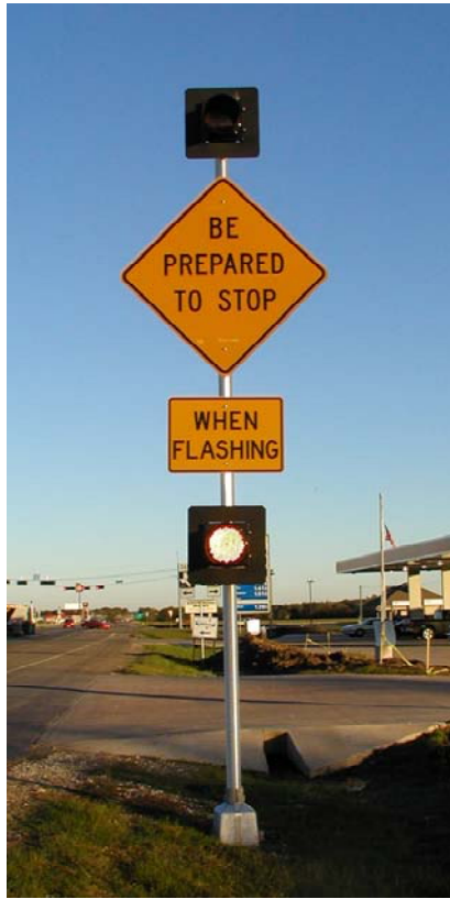
Figure 3. AWEGS Sign on a Single-Lane Approach.
