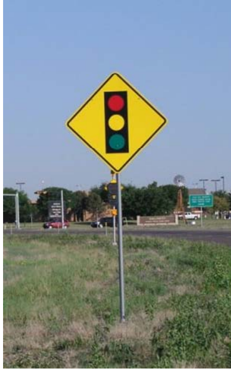
Figure 6. Signal Ahead Sign (W3-3) without Beacons.
