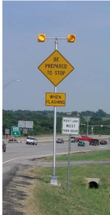
Figure 8. AWEGS Sign with the Beacons on Top.
