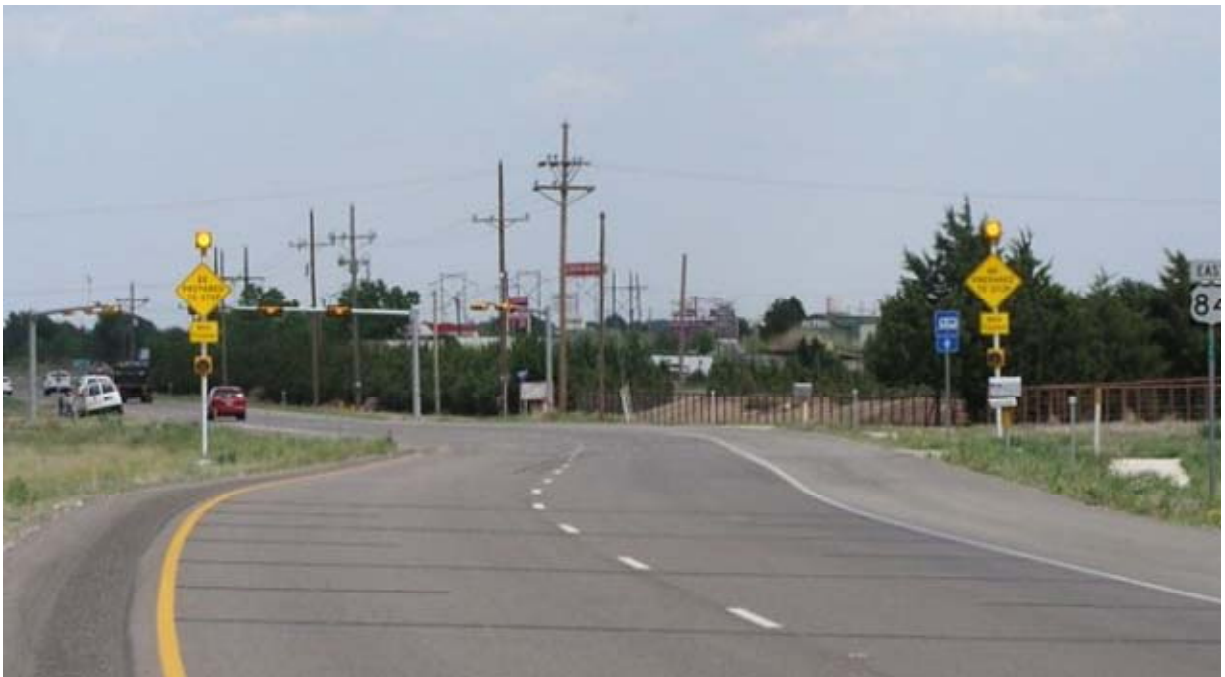
Figure 4. AWEGS Signs on a Two-Lane Approach.
