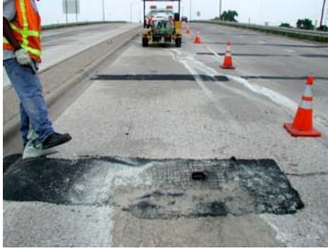
Figure 5.14 Highway 77 at Waco District
