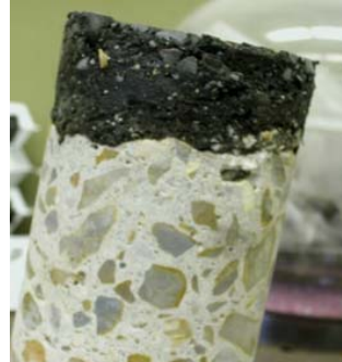
Figure 5.10 Core Taken from Location 8
