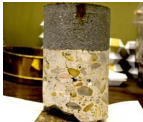
Figure 5.3 Core Taken from Location 2
