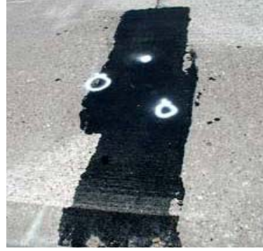
Figure 5.15 Patching Area with Fibrecrete
