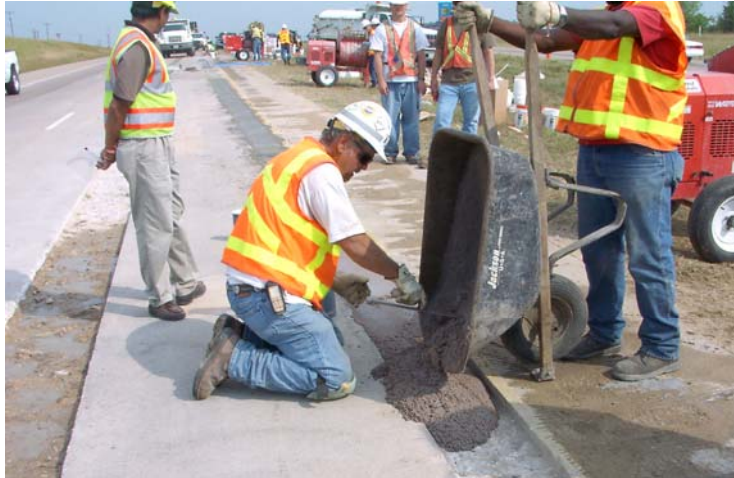
Figure 5.20 Placement of FlexPatch by Crews in Ft. Worth
