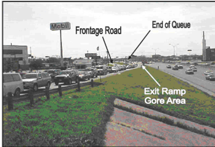
Figure 6-10. Plan View of Exit Ramp Spillback at Case Study Site 11.
