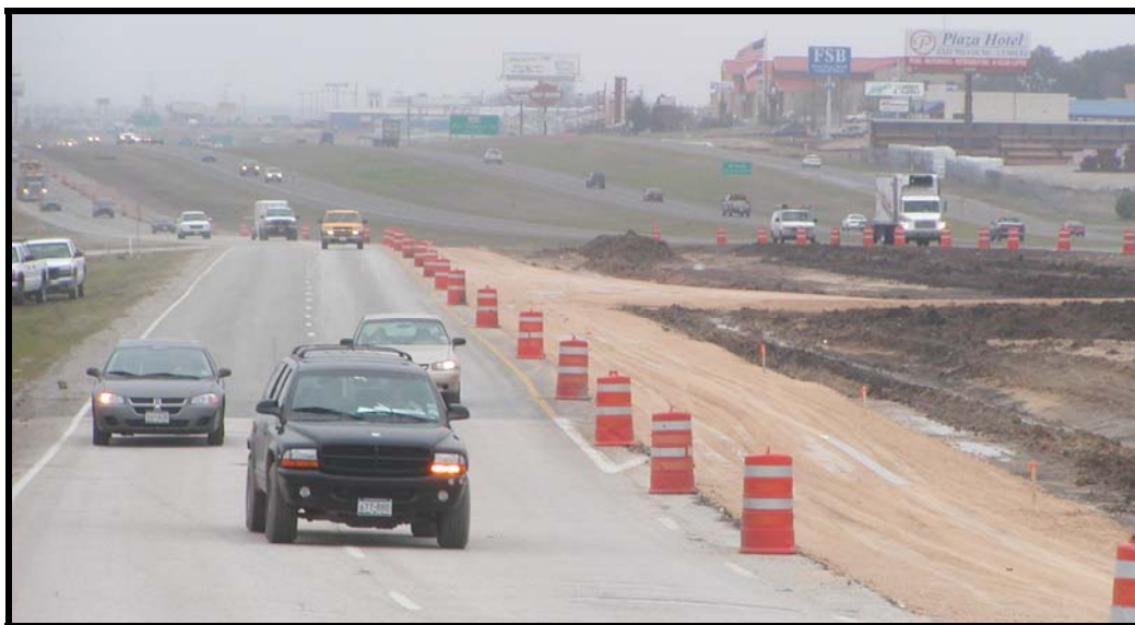
Figure 6-21. Picture of Construction of New Frontage Road Auxiliary Lane.
