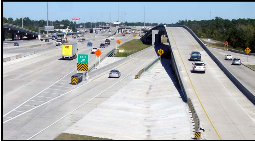
Figure 6-17. Braided Ramps in Houston, Texas.
