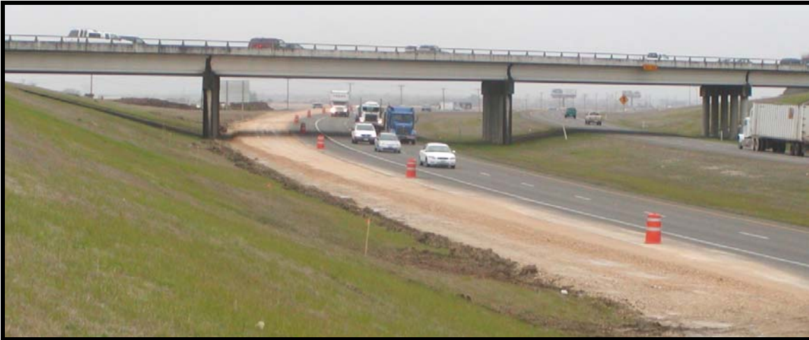
Figure 6-20. Picture Showing Construction of New Auxiliary Lane on Freeway Main Lanes.
