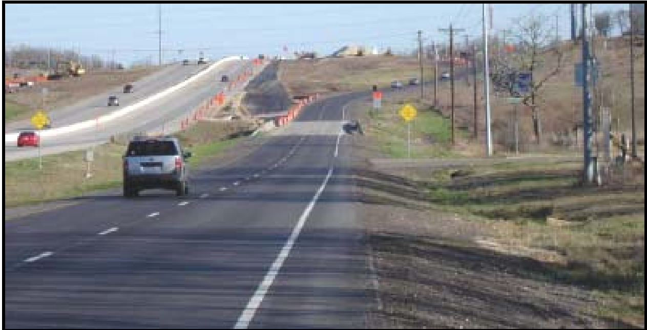
Figure 6-34. Evaluation of Frontage Road Operations is Important to Project Success.
