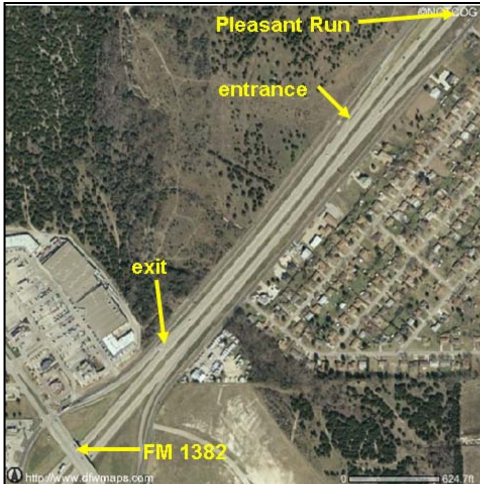
Figure 4-6. Aerial Photograph of Site 5 – US 67 in Cedar Hill (5).
