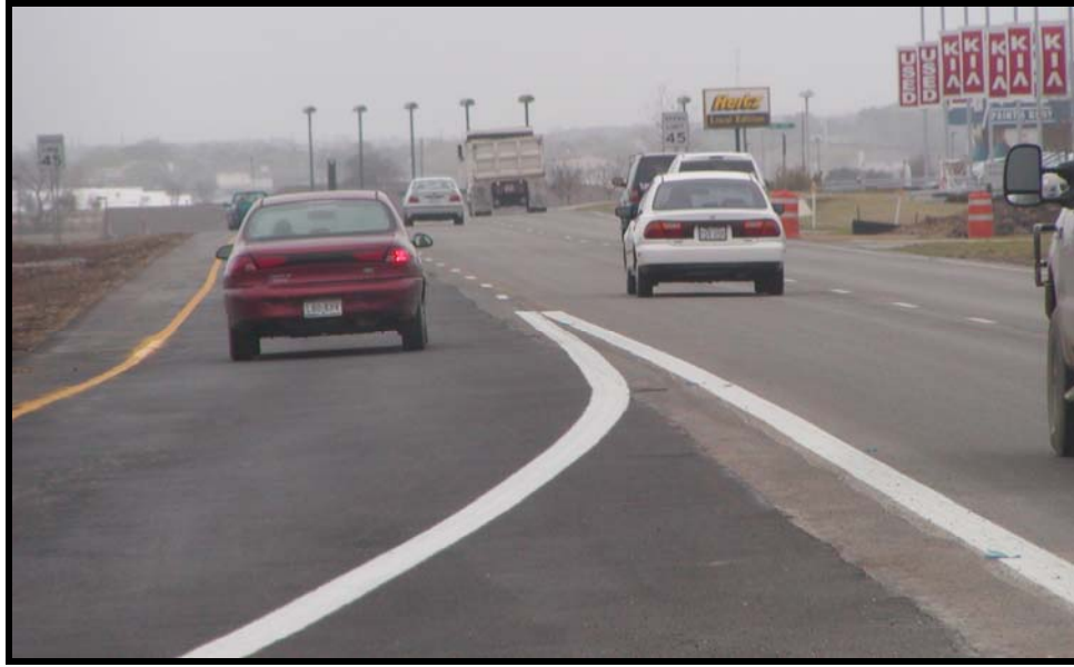
Figure 6-22. Frontage Road Auxiliary Lane.
