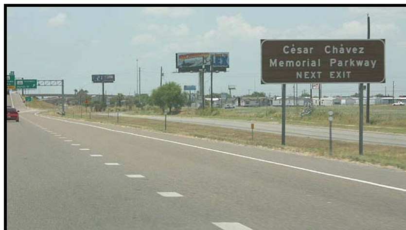
Figure 6-19. Freeway Auxiliary Lane.
