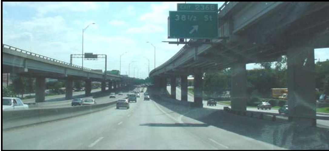
Figure 4-7. Picture of IH 35 Lower Level in Austin.
