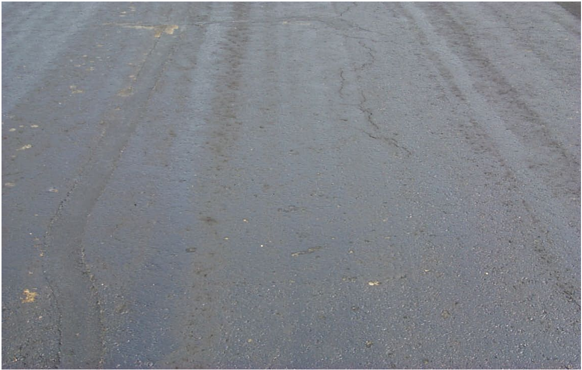
Figure 1-8. Sealed Aged Pavement.
