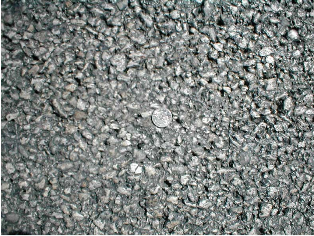
Figure B-11. Abilene, SH 36 L1, MS-2 Treatment Close-up (2006).
