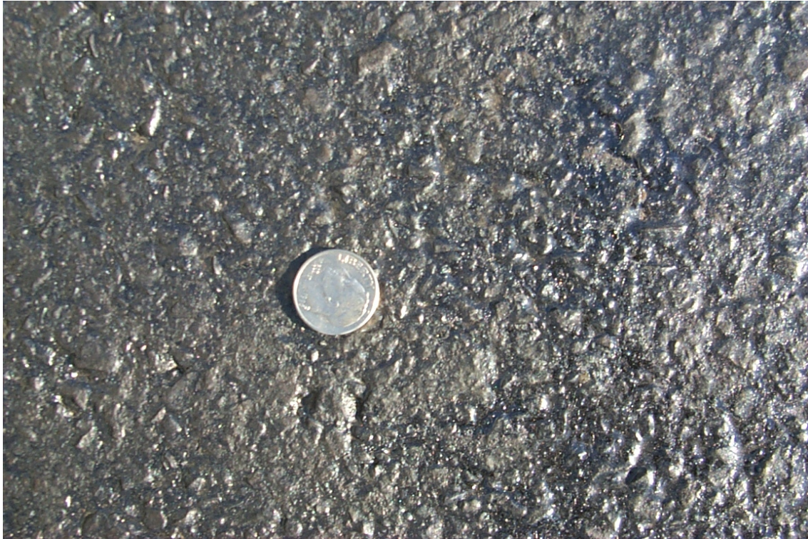
Figure B-39. Jacksonville Airport, Treated 2004 Close-up (2004).
