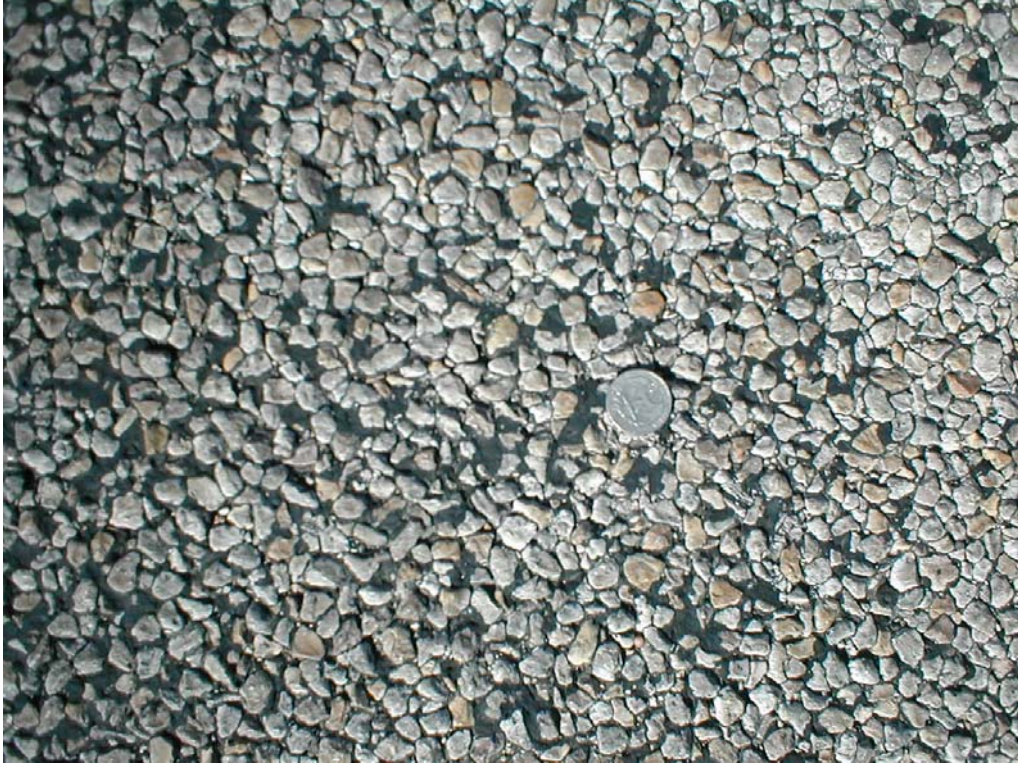
Figure B-45. Odessa Westbound Frontage Road, SH191, Treated 2002, Close-up (2006).
