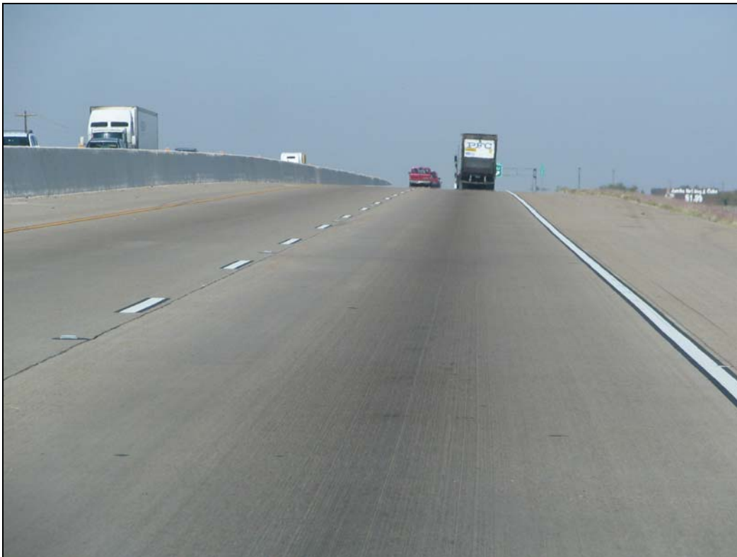
Figure 19. Bordered Contrast Markings, Skip and Edge (Waco, Texas).
