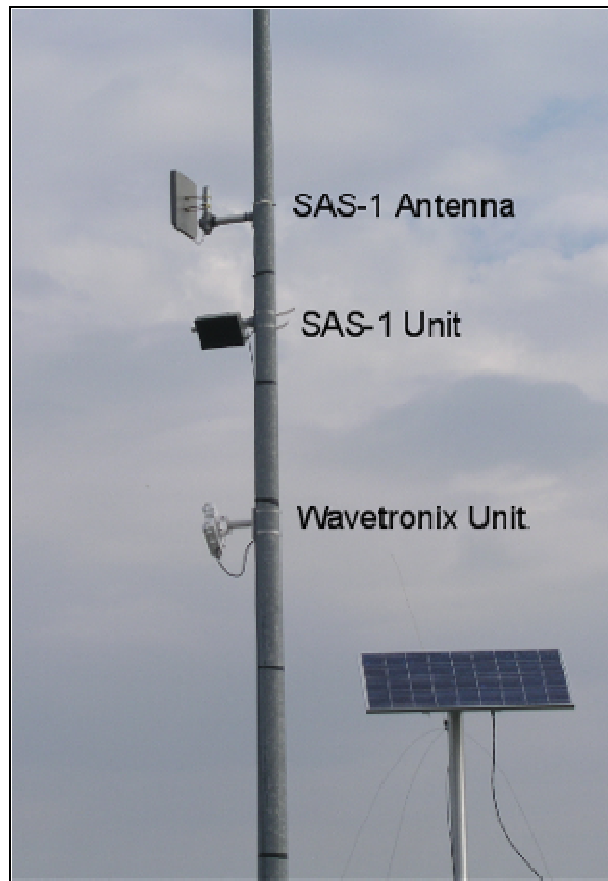
Figure 7. SAS-1 and Wavetronix Detectors.
