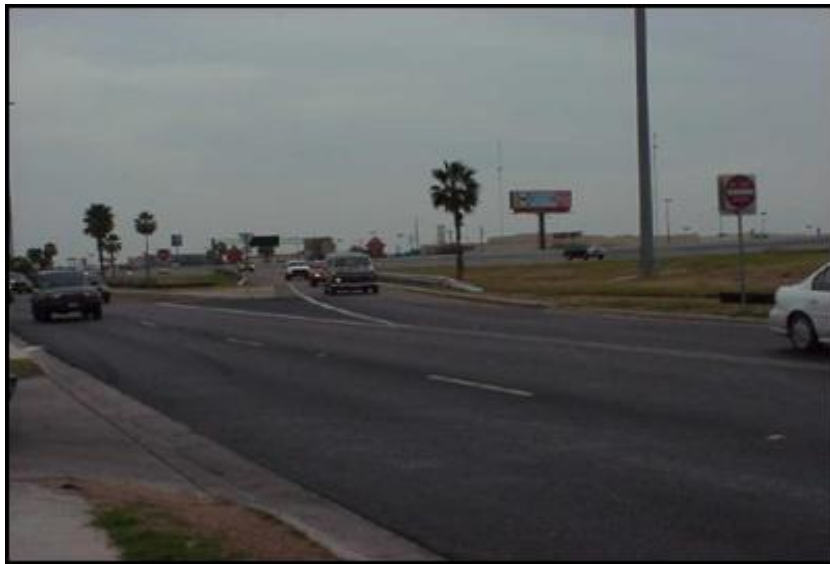
Site 7: Northbound I-35 at Mann Road Exit Laredo, Texas
