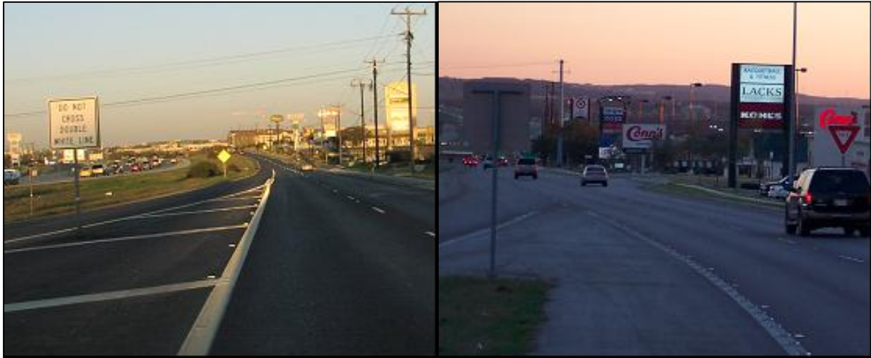
Figure 5. Example of Variations of Merge Treatment Application with Short Auxiliary Lane Provision for Exiting Traffic.
