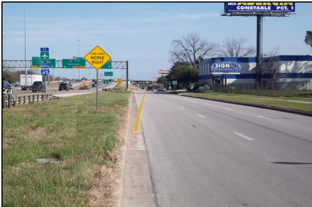
Figure 3. Example of Preferred Treatment with Frontage Road Lane Terminated Prior to Exit Ramp.
