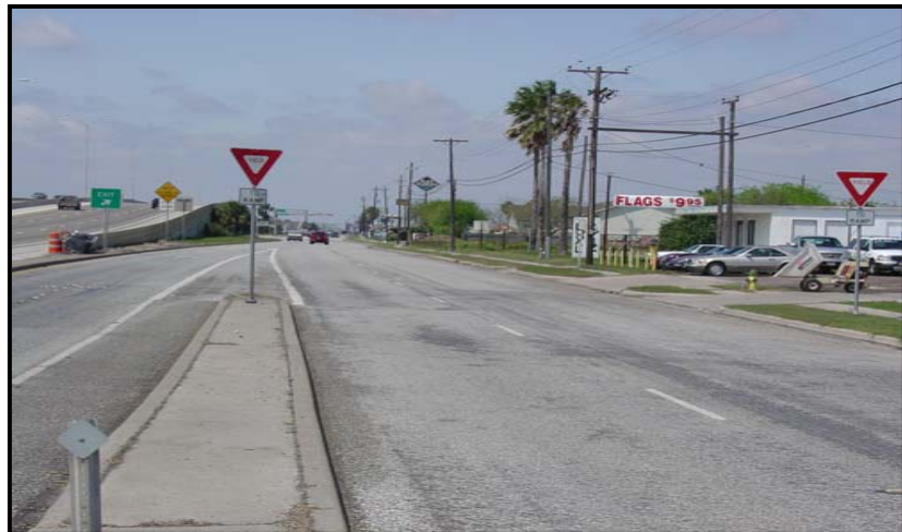
Site 5: Westbound SH 358 at Rodd Field Exit, Corpus Christi, Texas
