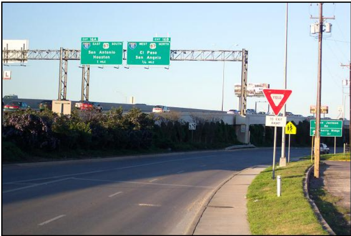
Figure 6. Example of the Use of Both a YIELD Sign and a Double White Line.
