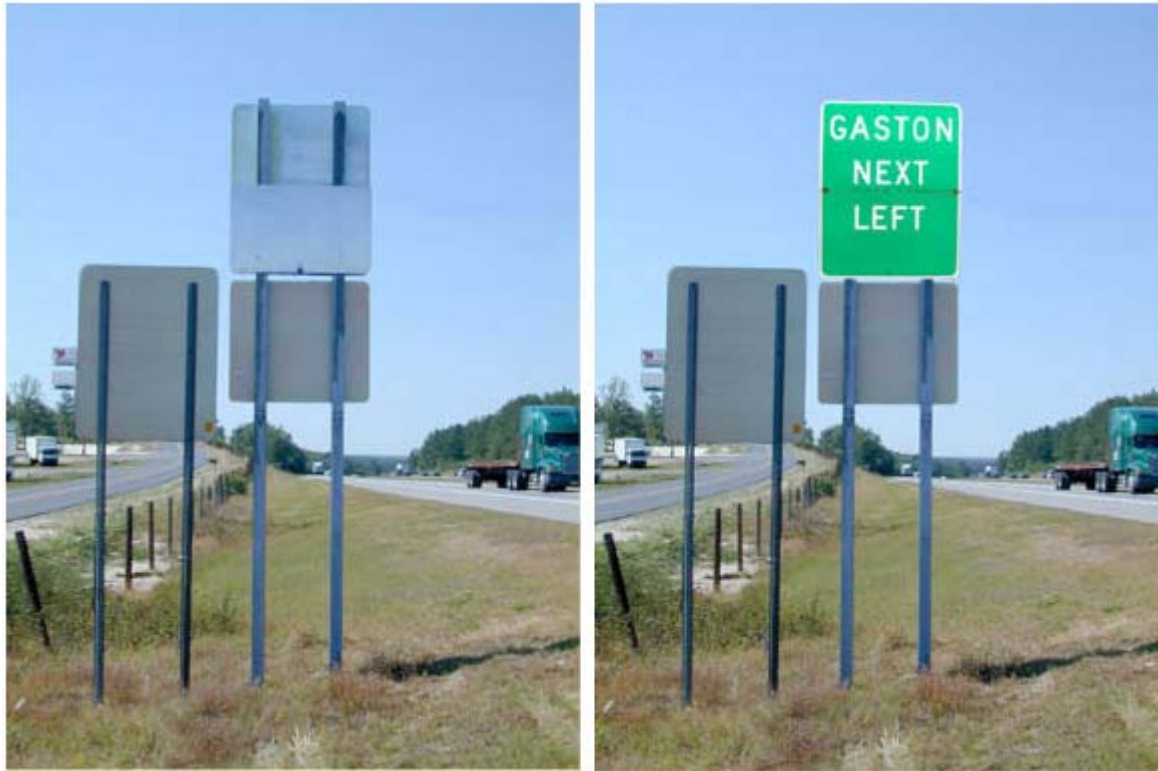
Figure 6. Flip-Down Sign on Contraflow Route in South Carolina ( 18 ).
