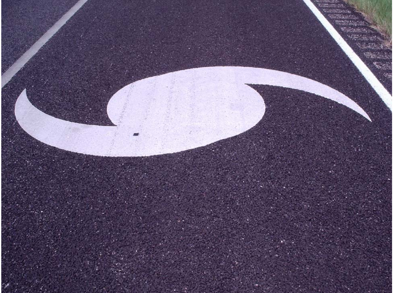
Figure 8. I-37 Emergency Shoulder Lane Pavement Marking.
