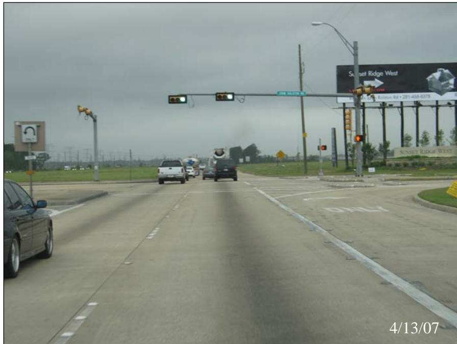
Figure 7-3. Typical Intersection Approach (Sam Houston Parkway, Northbound at John Ralston Road).
