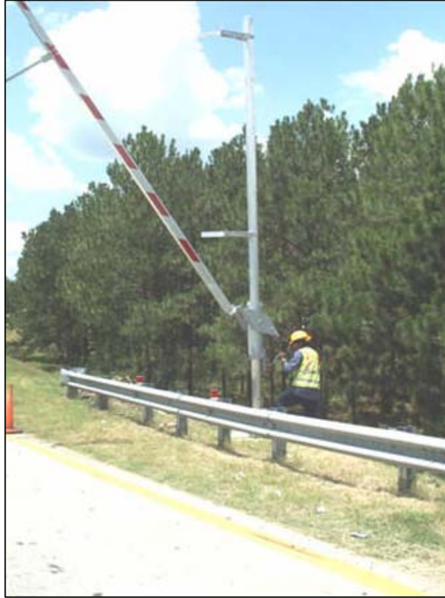
Figure 9-1. Contraflow Ramp Drop Gate Installation (27).
