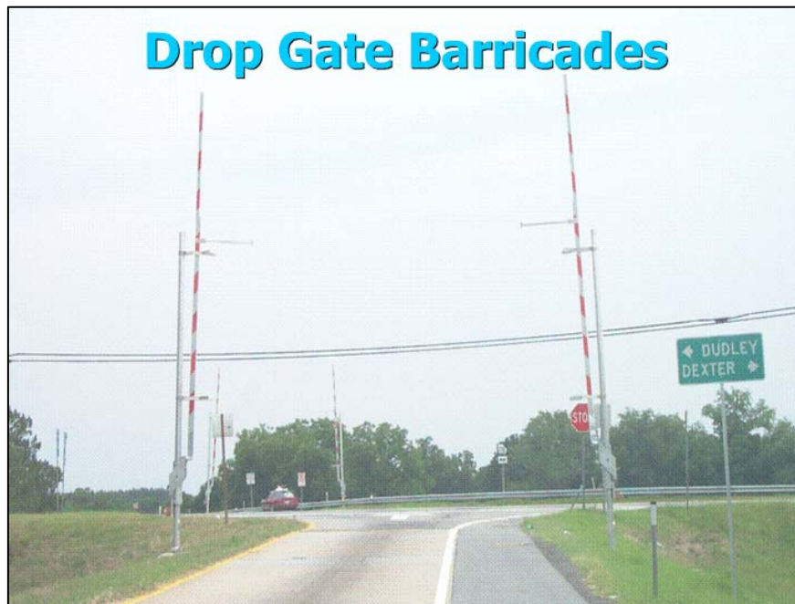
Figure 9-2. Georgia DOT's Drop Gate for Contraflow Ramps (27).
