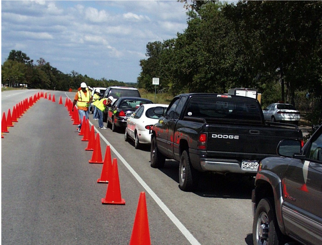
Figure 8. Typical Blocked Lane Configuration.
