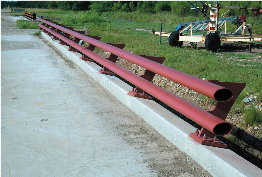
T77 Bridge Rail Prototype Installation.
