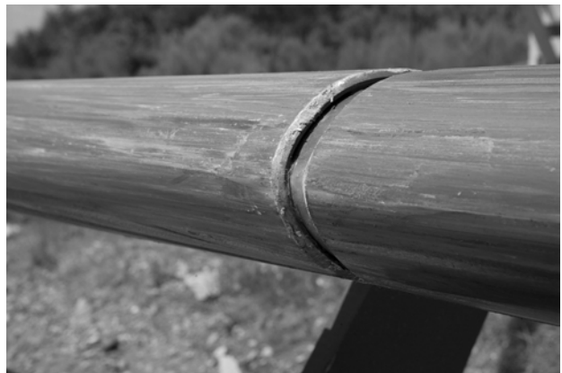
Figure 18. Installation After Test 409260-1.
