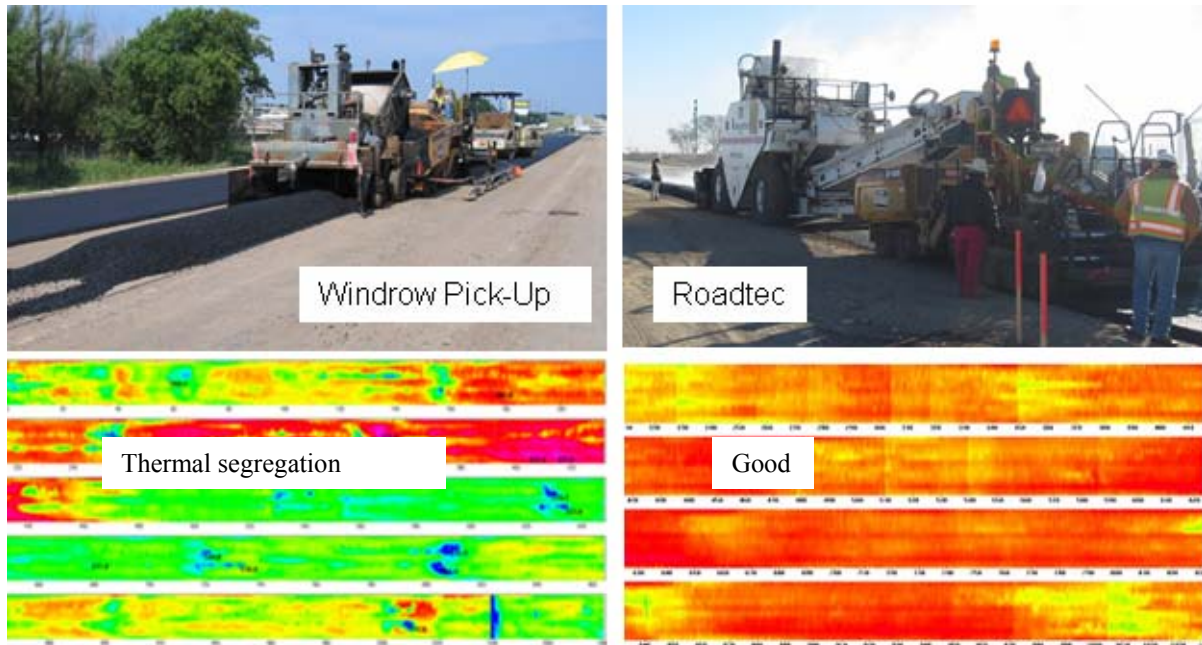
Figure E-1. Comparison of MTDs and HMA Mat Temperature Profiles on SH 114.
