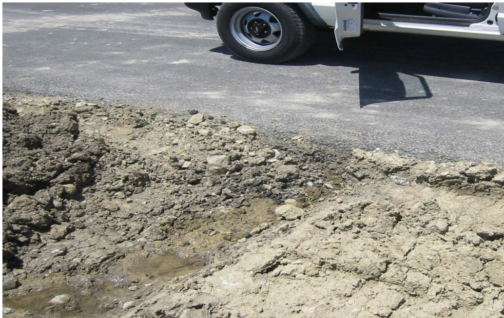
Figure 2-16. Water Draining from 1" SFHMAC into Relief Trench.
