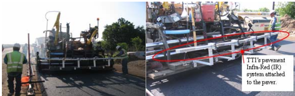
Figure 2-6. TTI's Infra-Red System and Mat Temperature Measurements.
