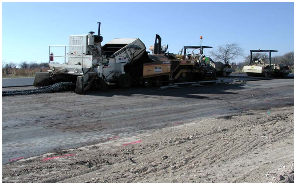
Figure 2-7. Roadtec Lay-Down Operation for RBL on Superpave Section (Dec 2003).
