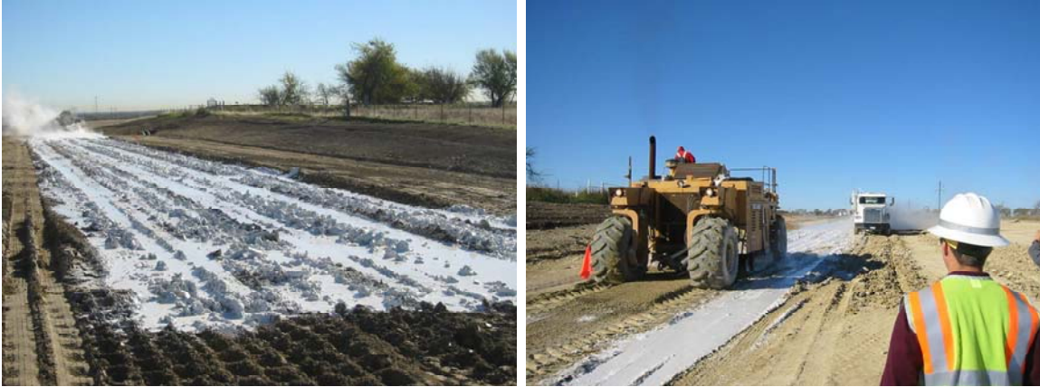
Figure 2-3. Subgrade Treatment with Lime Slurry.
