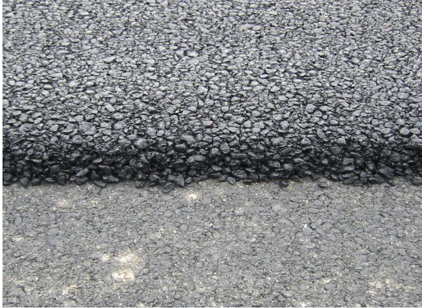
Figure 2-15. Coarse Nature of 1" SFHMAC Superpave Mix Used on SH 114.
