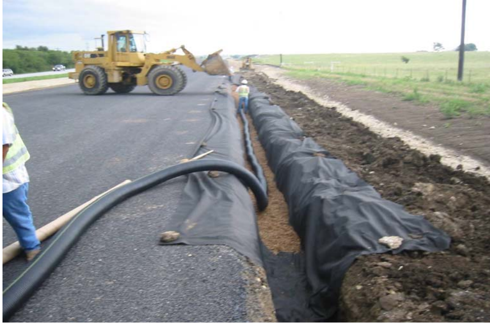
Figure 2-17. Edge Drain Installation on the Superpave Section.
