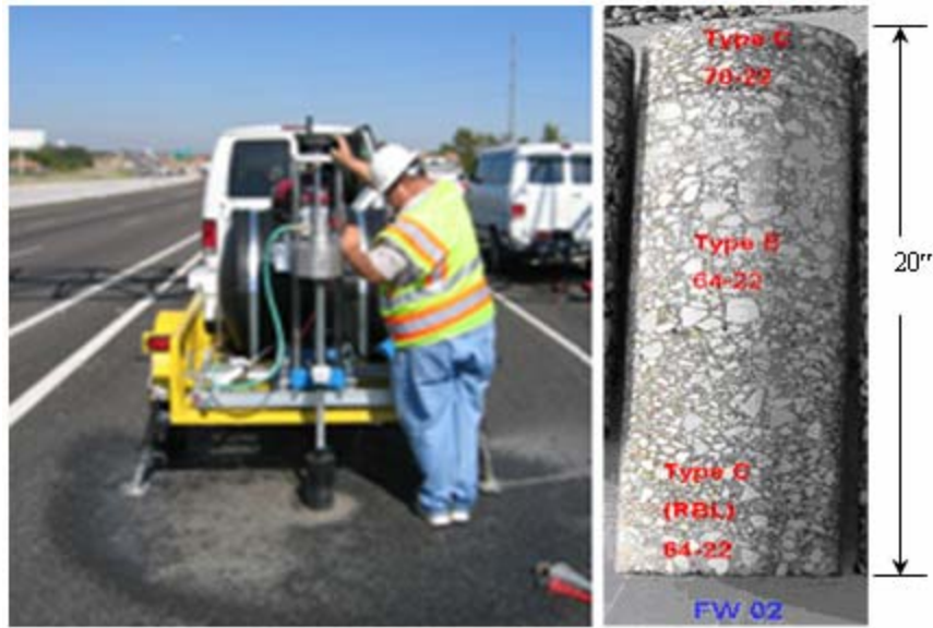
Figure 3-6. TTI's Coring Rig and Field-Extracted Core.
