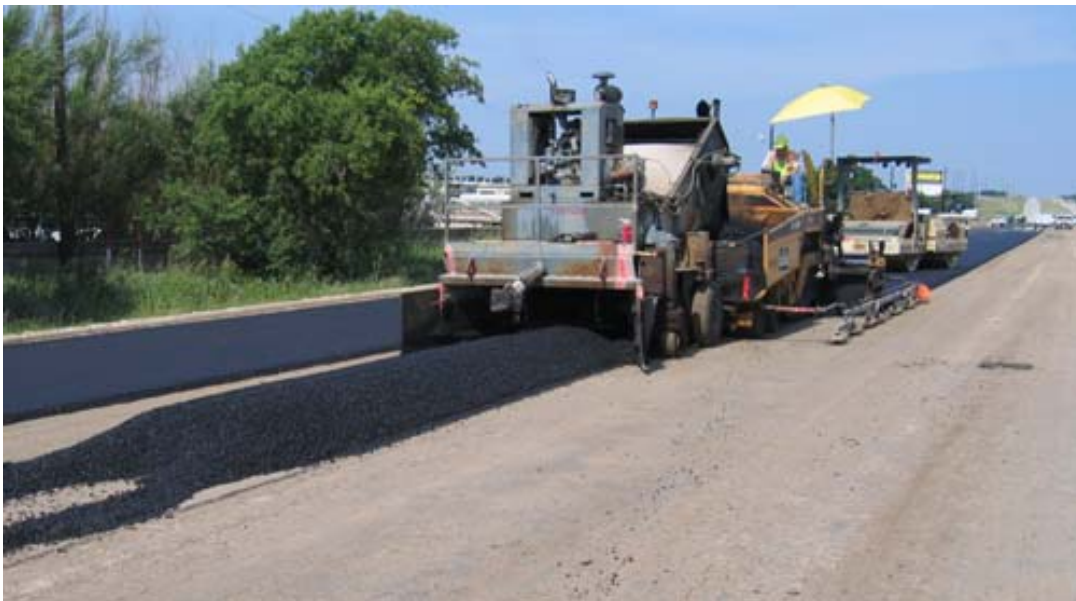
Figure 2-5. Windrow Pick-Up Setup for the RBL on the Conventional Section (May 2006).
