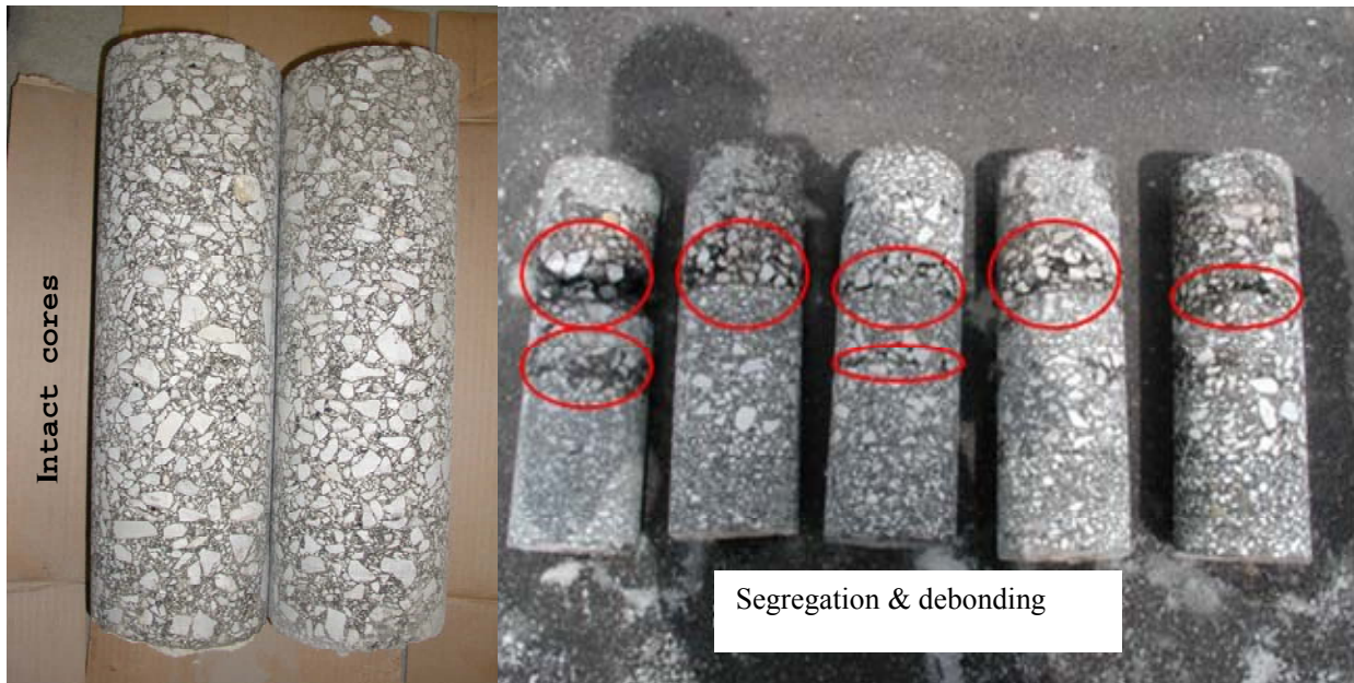
(c) IH 35 Hillsboro Project (3" compaction lift thickness)
