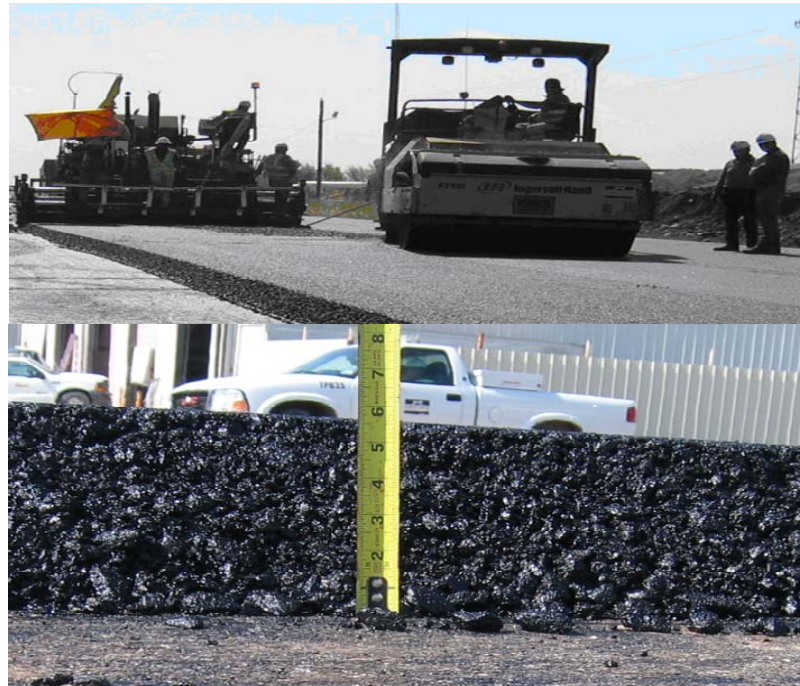
5" compaction lift thickness
