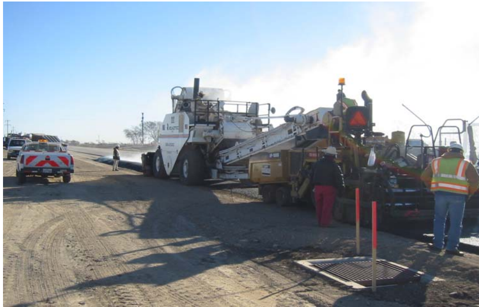
Figure 2-9. Revised Lay-Down Operation for All Subsequent Layers on Superpave Section.
