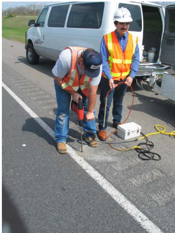
Figure 17. Temperature Probe Installation.
