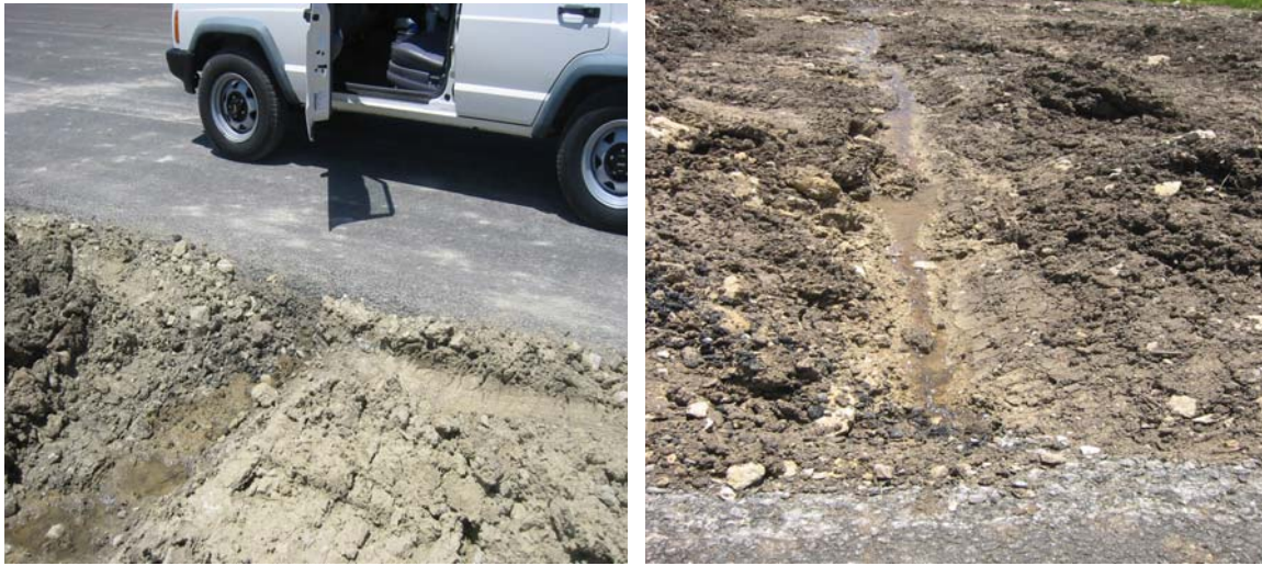
Figure 26. Releasing Trapped Water from the Stone-Filled Asphalt Layers on SH 114.
