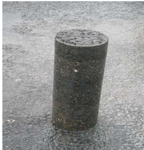
Figure 18. Intact Cores from the Gilbert Project in Laredo.
