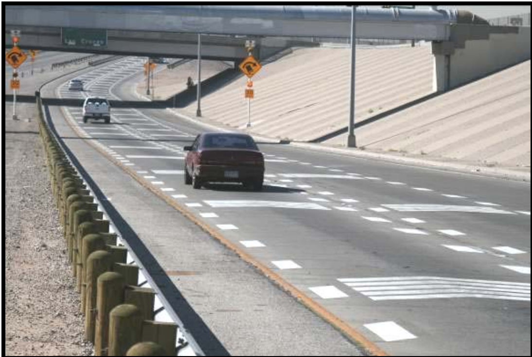
Figure 20. View of Chevron Markings with Existing Flashing Advisory Speed Warning Sign (30 mph).
