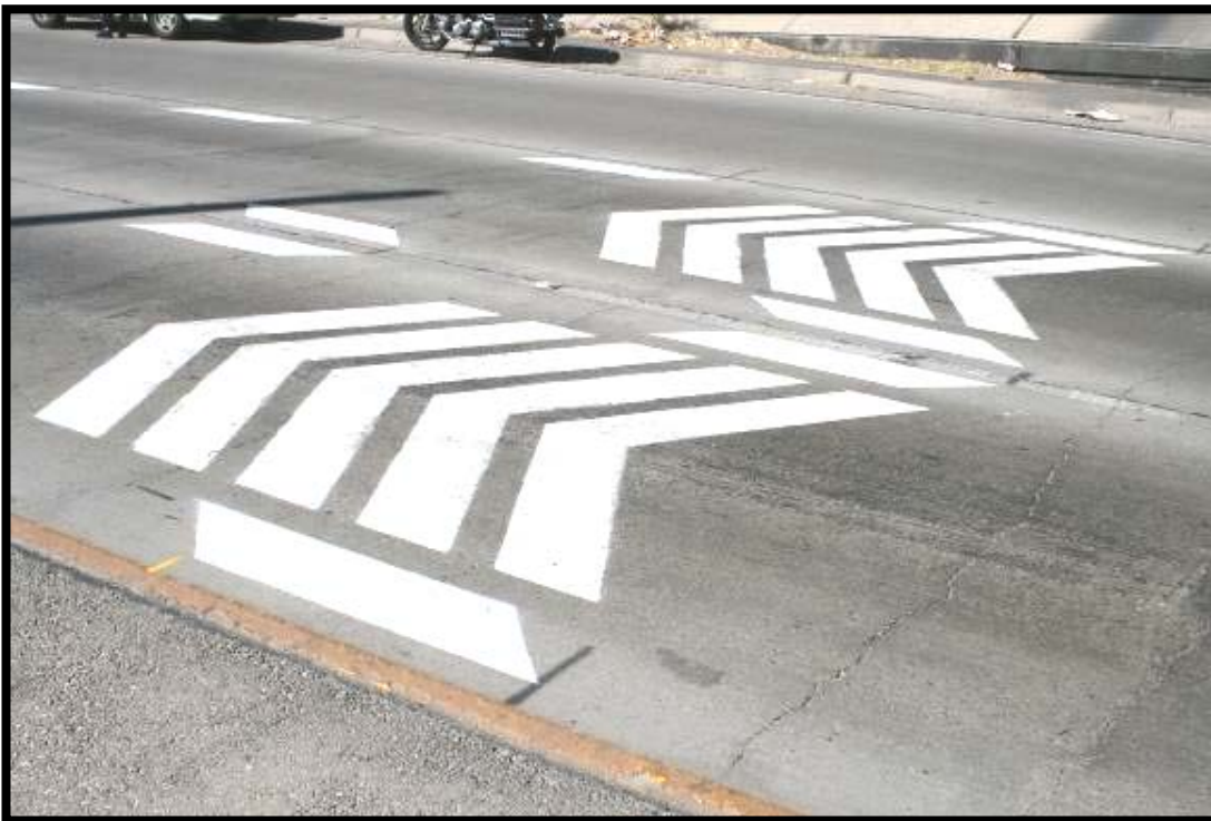
Figure 18. Closer View of Chevron Markings Implemented at Site.
