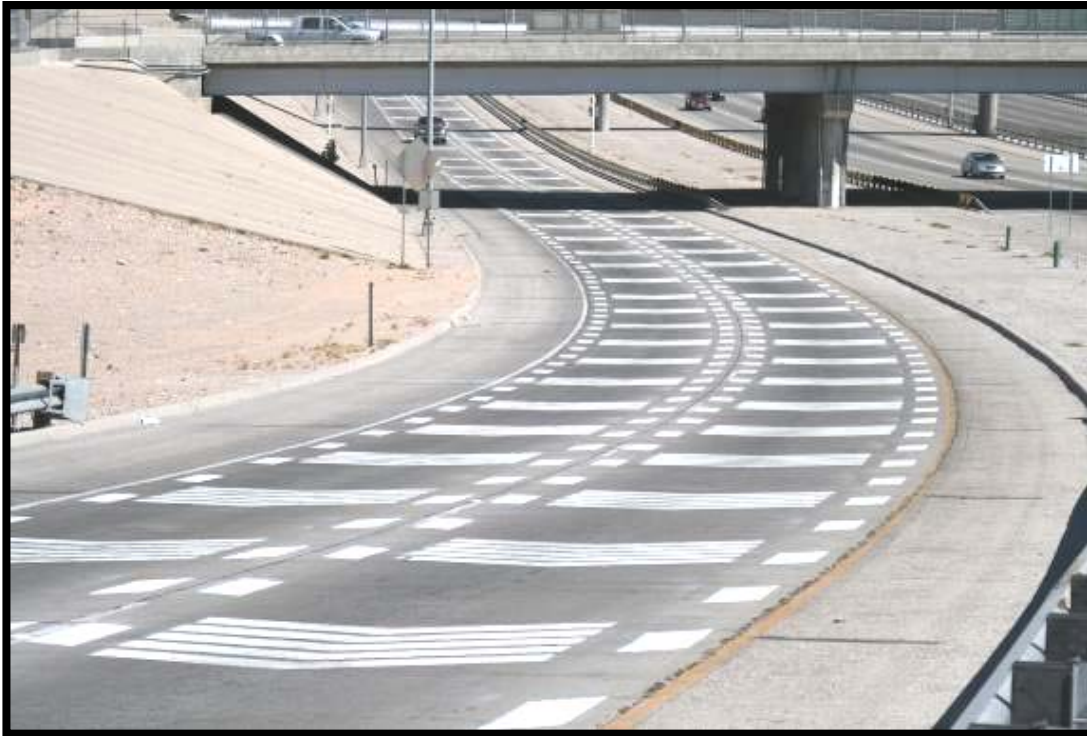
Figure 17. View of Chevron Pavement Markings Implemented on the Approach to the US 54 Westbound to IH 10 Westbound Freeway-to-Freeway Connector Curve.
