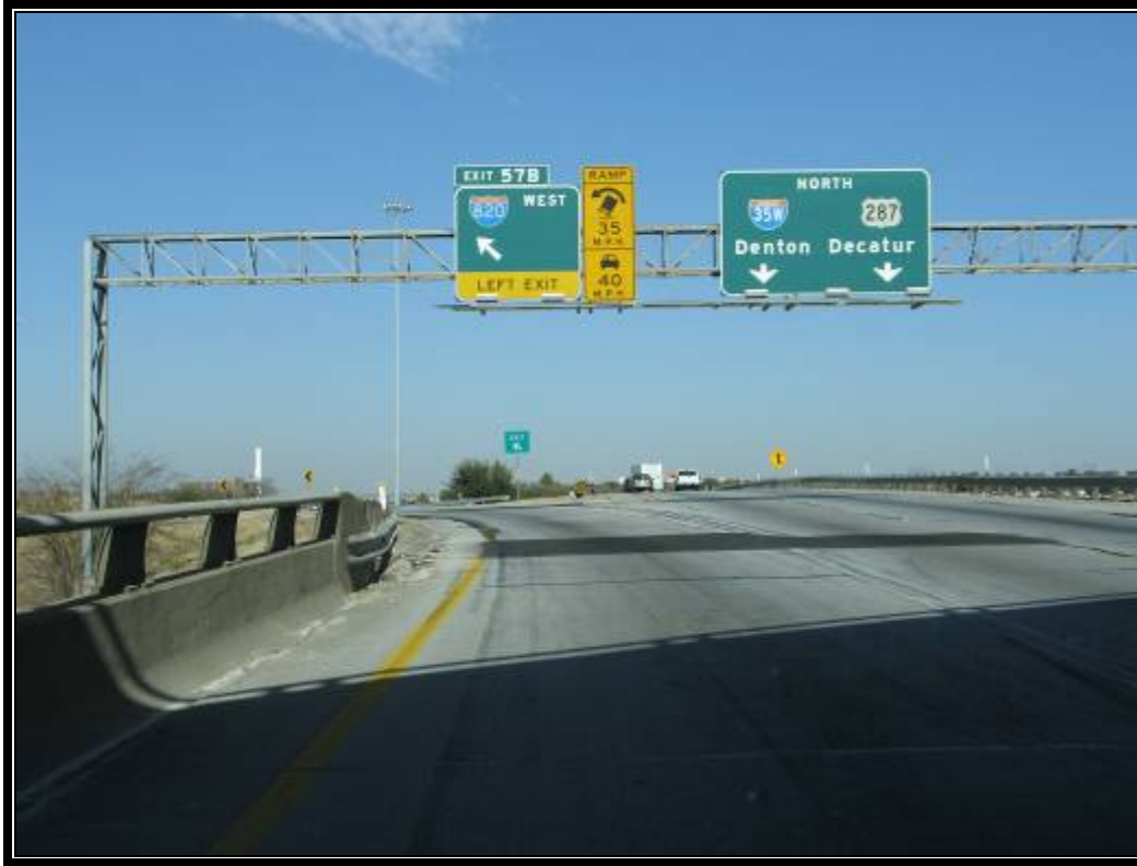
Figure 38. IH 35W Northbound to IH 820 Westbound (Fort Worth 1 – at PC, Overhead).
