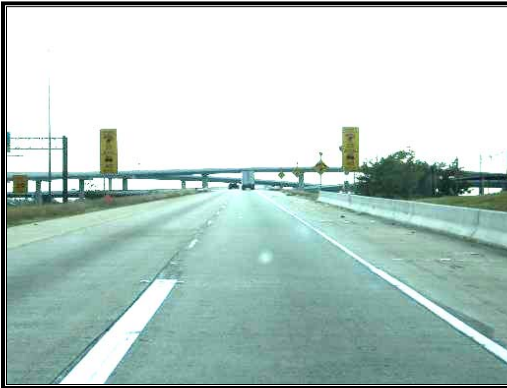
Figure 42. US 59 Southbound to IH 610 Eastbound (Houston 2 – at 500 feet upstream of PC).
