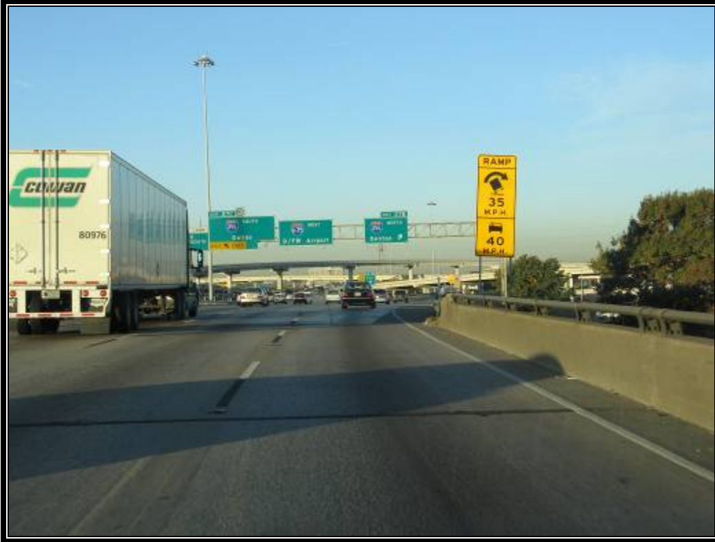
Figure 35. IH 635 Westbound to IH 35E Northbound (Dallas 3 – Upstream).
