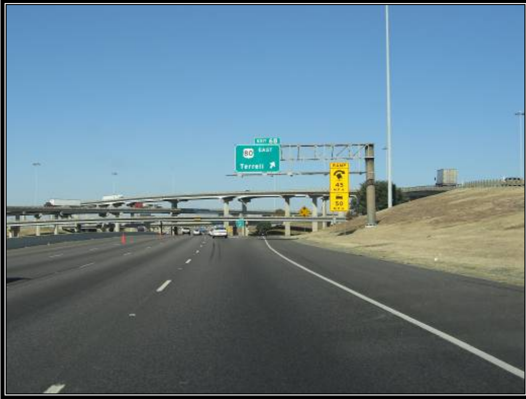
Figure 33. IH 635 Northbound to US 80 Eastbound (Dallas 1).
