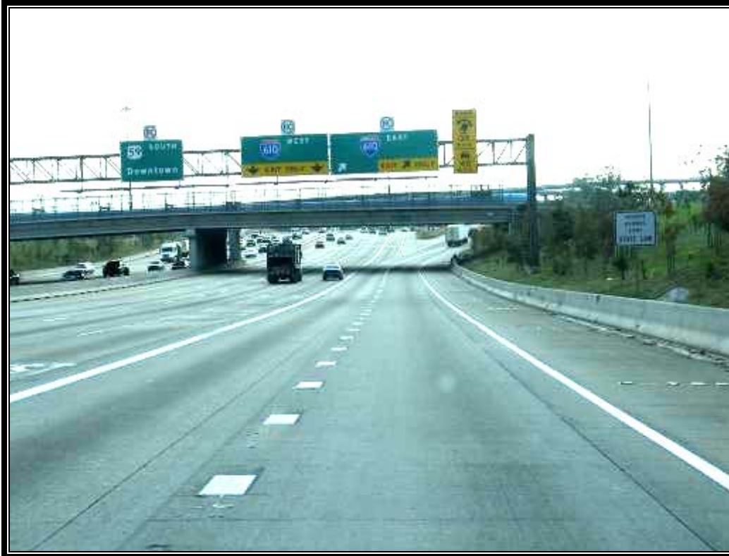
Figure 41. US 59 Southbound to IH 610 Eastbound (Houston 2 – Upstream Overhead).
